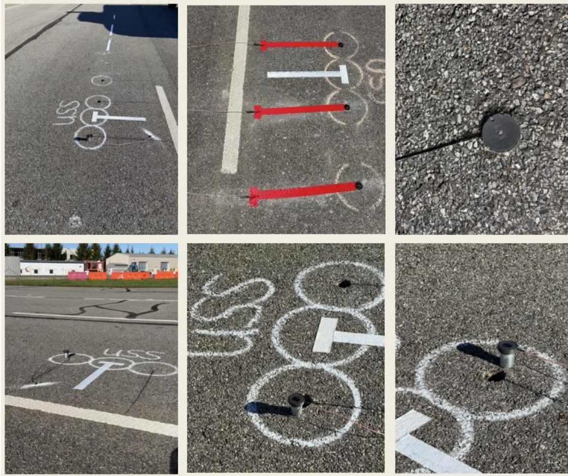
Figure 10. Geophones set up on the Surface Street section; red tape shows location of geophones; white tape shows location of LDV target points.
