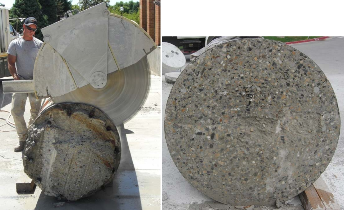
Figure 3. Saw-cut of 36 in. diameter column from Highland Drive Bridge.
