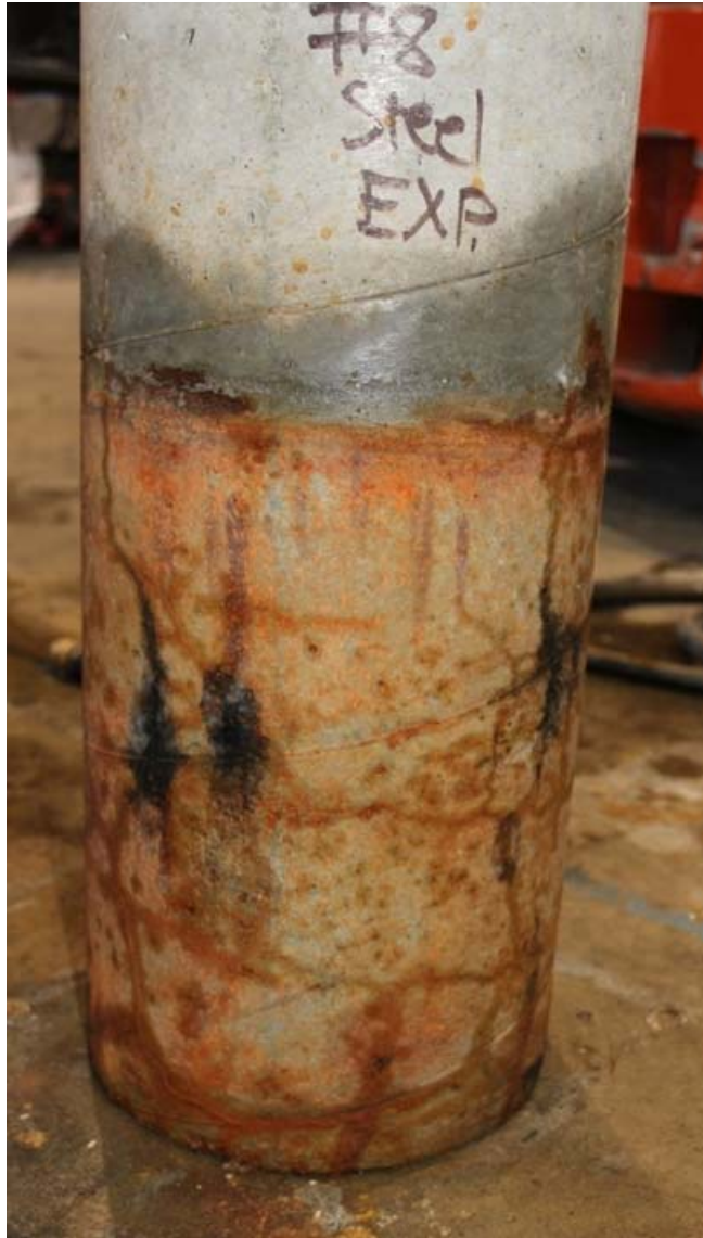
Figure 2. Corrosion deterioration of first small-scale steel reinforced column.
