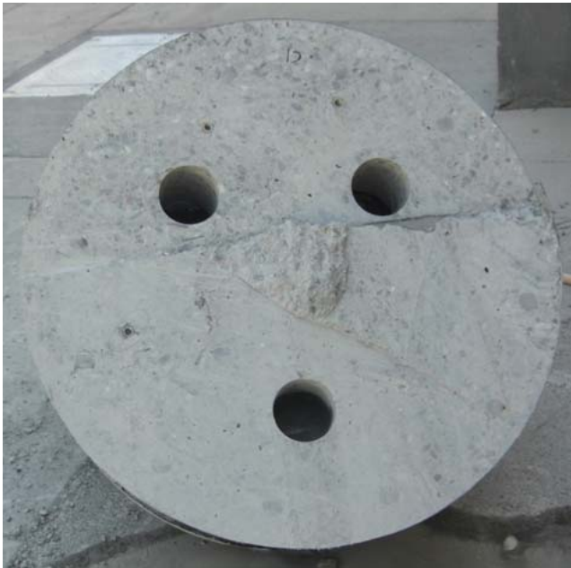
Figure 4. Concrete cores from cut-off column section.
