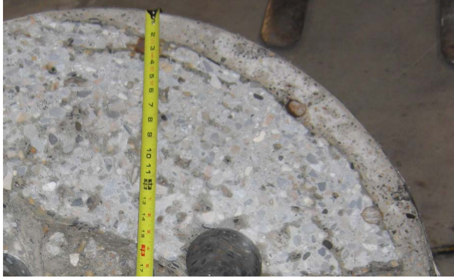
Figure 6. Replaced concrete around the perimeter of column section.
