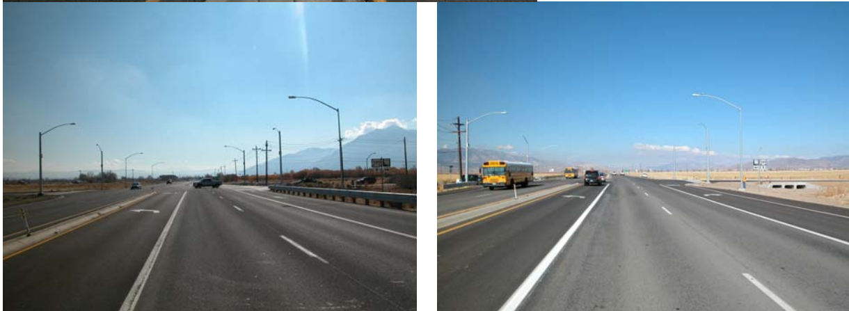
FIGURE 4-5 US 395 Turn Lanes on the North (left photo) and South (right photo) Approaches
