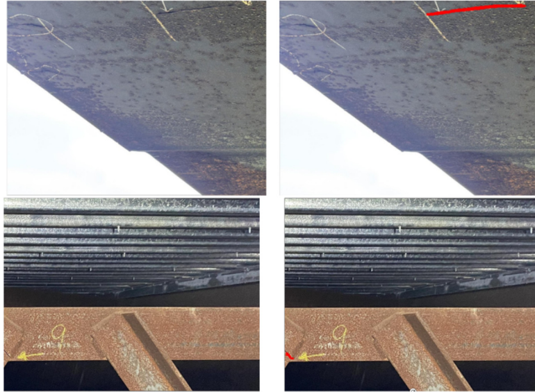
Figure 4. Example of crack segmentation results: original images (left) and model's output (right).
