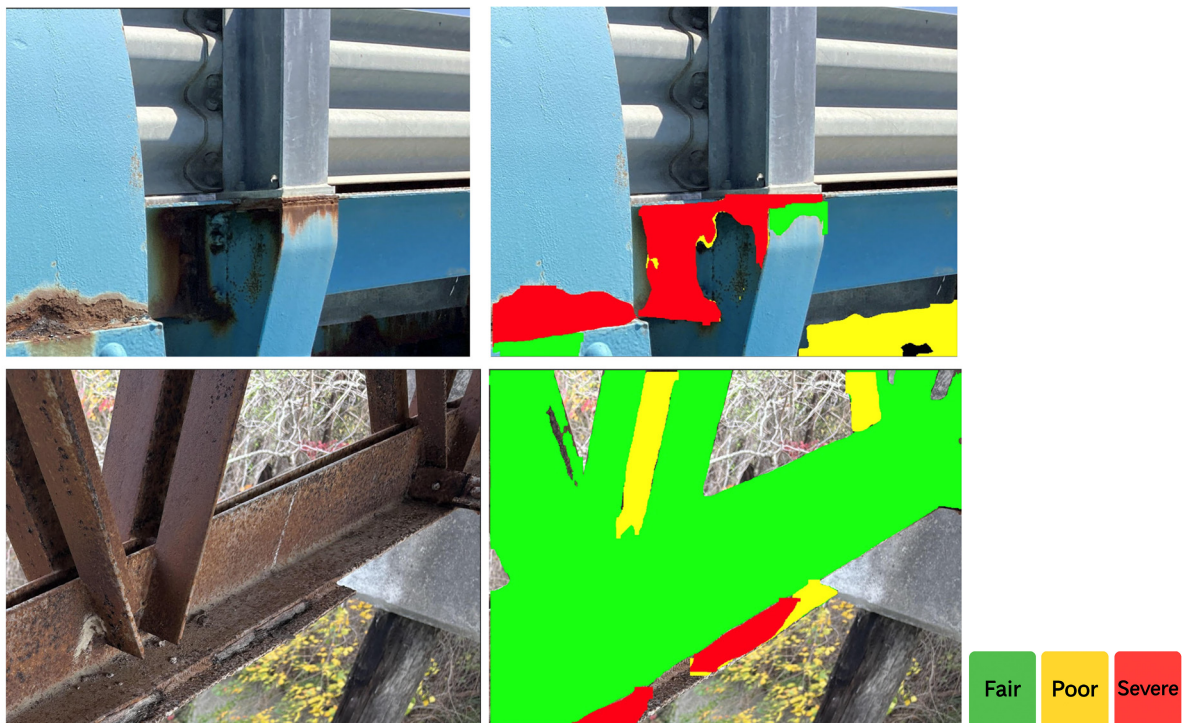
Figure 3. Example of corrosion segmentation results: original images (left) and model's output (right)
