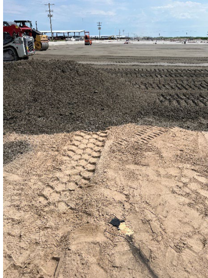
Figure 13. REBEL sensor in the roller-compacting concrete
