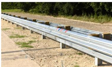
This project evaluated the W-beam median guardrail system with a rubrail mounted below the W-beam rail element on one side of the system. The median guardrail system was evaluated using MASH TL-3 criteria for longitudinal barriers. MASH Tests 3-11 and 3-10 were performed. The median guardrail system with the rubrail passed both tests and is considered MASH TL-3 compliant.
