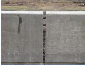
Concrete bridge rail systems tested and evaluated according to MASH typically include joint openings between ½ to 2 inches. Bridge rail systems with larger joint openings have not been evaluated according to MASH. Guidelines were developed for MASH compliant joint opening widths and solutions to protect joint openings that are not MASH compliant.
