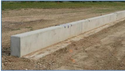
Low-profile barriers can offer improved sight distance and provide a barrier option that can more unobtrusively integrate into adjacent urban surroundings. Florida DOT desired to develop a permanent, cast-in-place, low-profile concrete barrier that meets MASH TL-2 criteria. Finite element modeling and simulation was used to recommend a 20-inch-tall, vertical-profile, concrete barrier for full-scale
