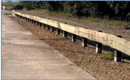
Connecticut DOT uses steel-backed timber guiderail as an aesthetic barrier system on the scenic Merritt Parkway. A MASH compliant version of this rail was needed for inclusion in CTDOT's standards. The existing design installed over a 4-inch curb did not meet MASH criteria for Test 3-11. A modified version of the steel-backed timber guiderail was evaluated and determined to be MASH TL-3 compliant. The modification involved a reduction in post spacing from 10 ft to
