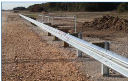
In this research, the Long-Span Guardrail was evaluated with a fall-protection fence installed behind it. This fence is installed on concrete culverts used for fish passages crossing state highways in Washington. The design was evaluated through finite element modeling and simulation, followed by full-scale crash testing. The Long-Span Guardrail installed in front of the fall-protection fence met the performance criteria for MASH TL-3 for longitudinal barriers.
