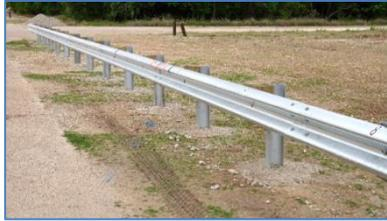
This project's objective was to determine the minimum length of an MGS without downstream anchorage required to provide MASH compliant redirective behavior. Computer simulations were performed to predict the minimum length-of-need prior to crash testing. MASH Test 3-11 resulted in the W-beam rail pulling off the posts, which violated the objective of the project.
