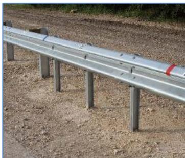
This project developed a transition from the weak-post W-beam guardrail to strong-post MGS guardrail system. It utilized reduced post spacing of the S3×5.7 weak steel posts to achieve a stiffness similar to the MGS with the standard post spacing. The transition system met MASH TL-3 performance criteria.
