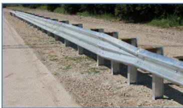
In this research, MASH-compliant thrie-beam median guardrail and thrie-beam roadside guardrail systems were developed using simulation and crash testing. The design of these guardrail systems used only the standard MGS components with the exception of the thrie beam rail element. Based on the full-scale tests and impact simulation analyses performed, it was concluded that both systems meet MASH TL-3 evaluation criteria for longitudinal barriers.
