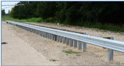
The objective of this research project was to evaluate reduced post spacing variations of the Midwest Guardrail System (MGS) for MASH compliance. A quarter-post spacing system successfully met MASH evaluation criteria for Tests 3-11 and 3-10. A modified half-post spacing system with shortened blockouts successfully met MASH evaluation criteria for Test 3-11. A transition between full- and quarter-post spacing
