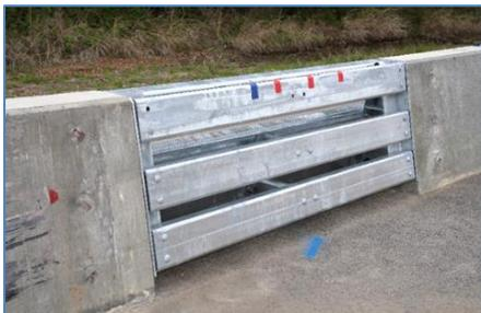
This research redesigned and tested a new tubular barrier gap rail system to use for a 36-inch-high single slope barrier. Report of an earlier phase of this research is available at the Pooled Fund's [website](#). This gap rail is needed in instances where manholes and other features located along the barrier alignment need to be accessed. The new gap rail design was attached flush with the concrete single slope barrier on each side. The gap rail design was tested with the small car
