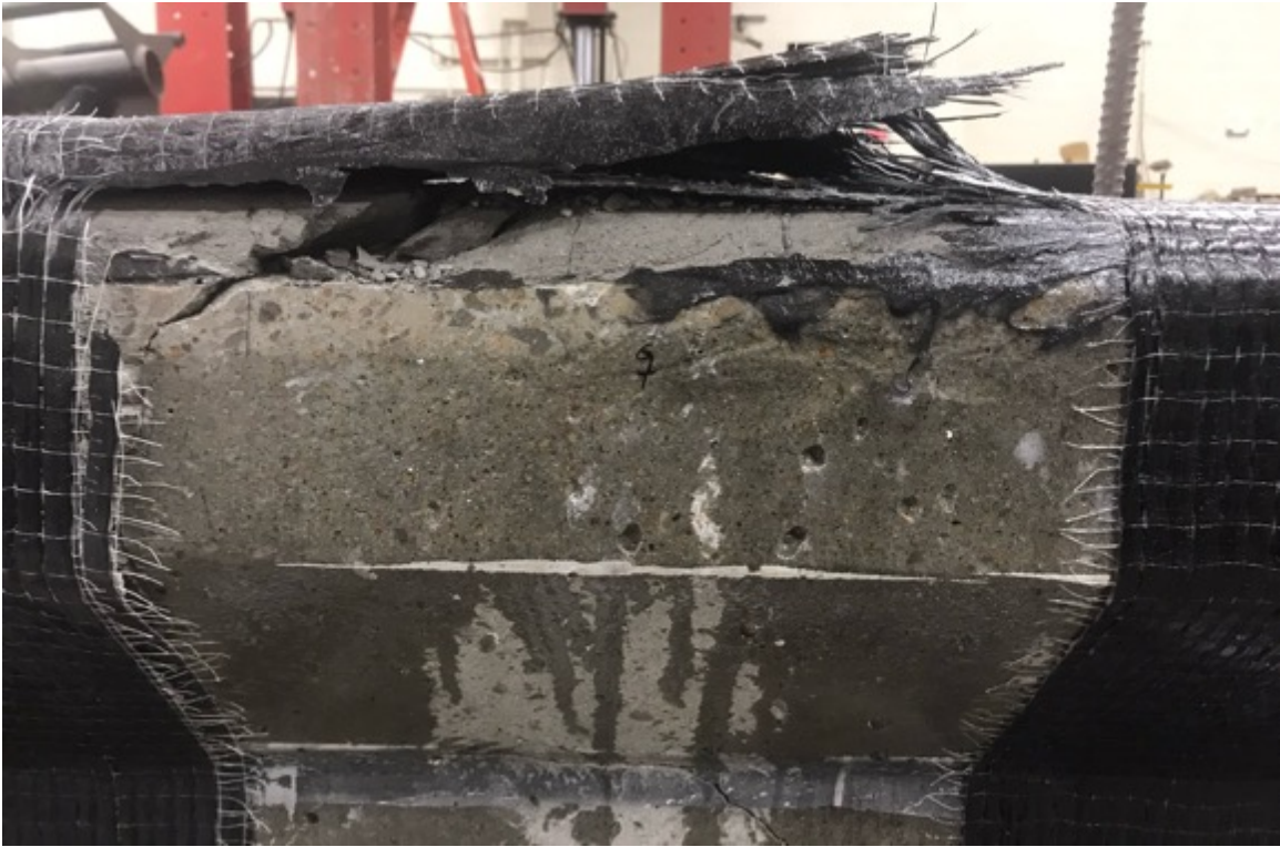
Fig. 1: Steps to repair and test a girder having 33% loss of strands with CFRP.
