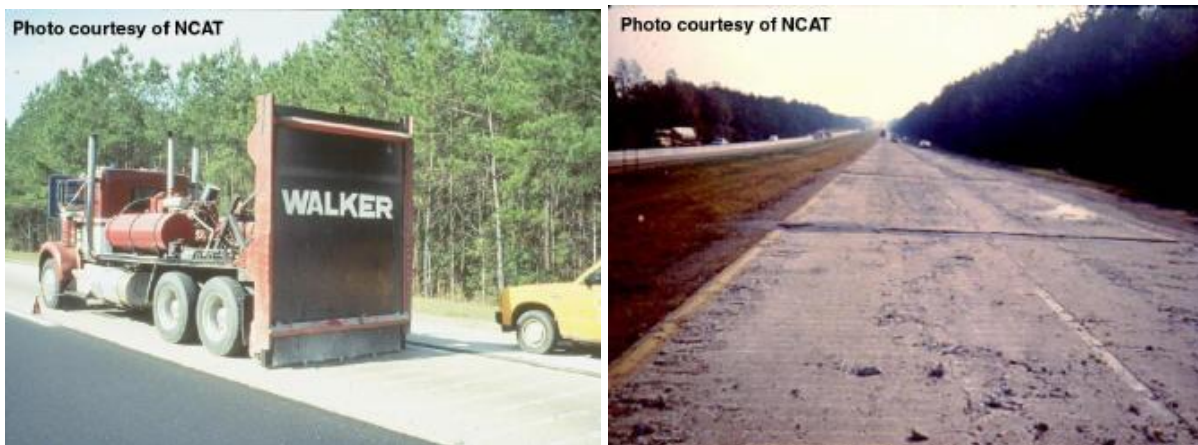
Figure 3.4. At left, guillotine hammer used for cracking and seating PCC; at right, PCC pavement after cracking and seating with guillotine hammer (WSDOT)
