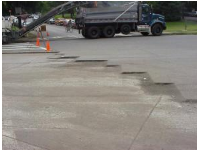
Figure 3.1. Milled road showing complete removal of the HMA overlay to expose the PCC slabs beneath (WSDOT).
