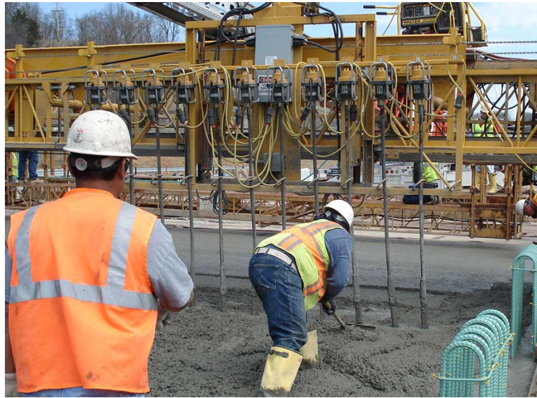
Fig. 5. 23 Gang vibrator system used for consolidation.
