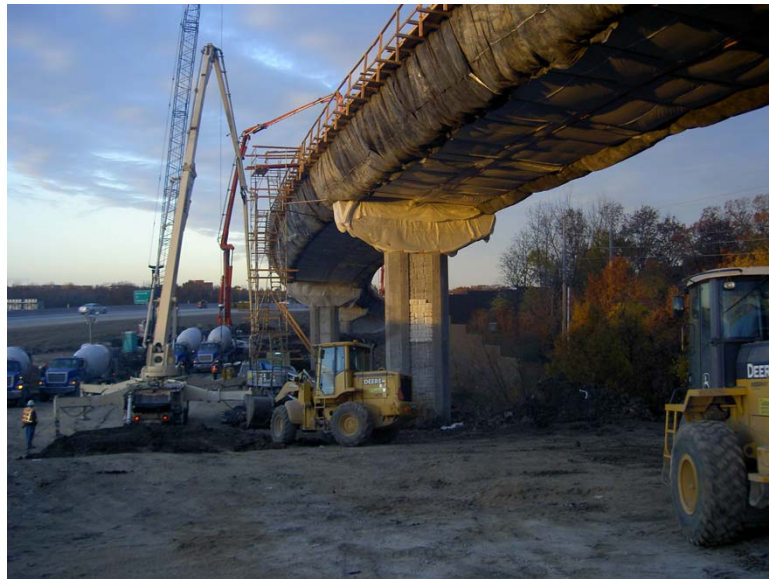
Fig. 5.34 Girders wrapped and heated on LC-HPC-5
