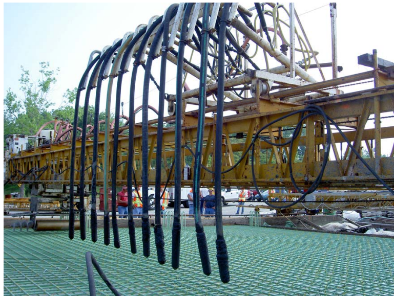
Figure 4.1 Vertically mounted internal gang vibrators.
