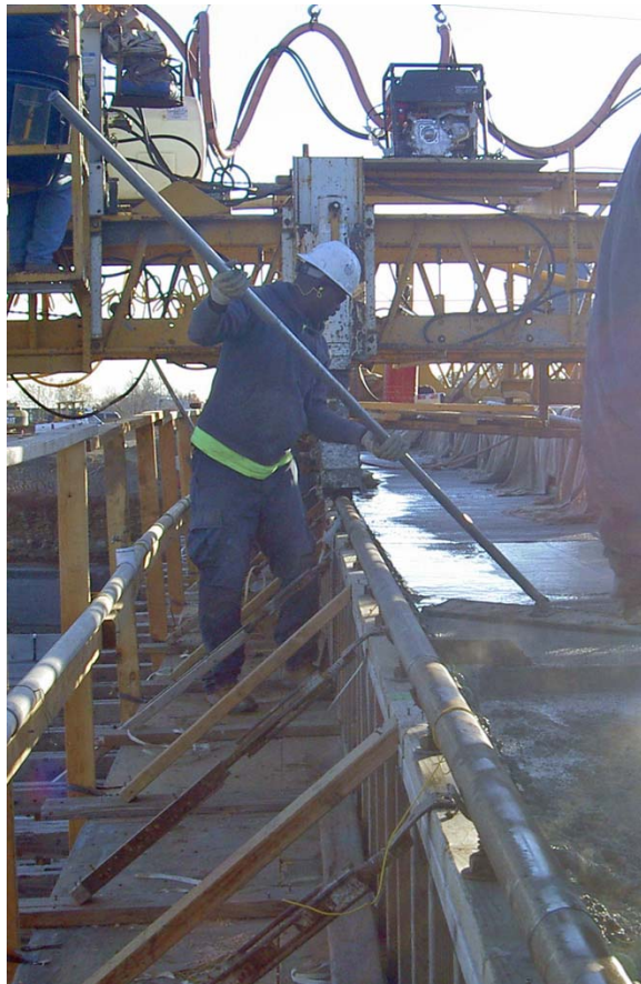
Fig. 5.33 Water worked into surface of the sidewalk
