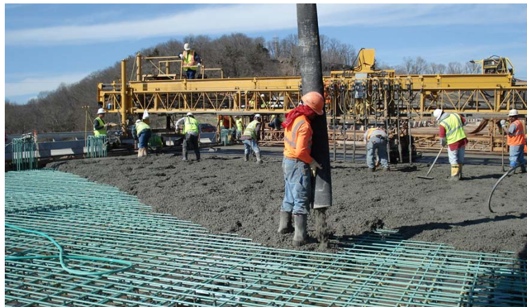
Fig. 5.22 Concrete placed in front of the finishing equipment at a skew
