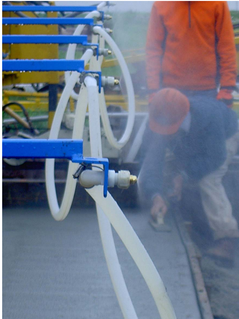
Fig. 5.16 Fogging system with flexible pipe - dripped water onto the deck surface
