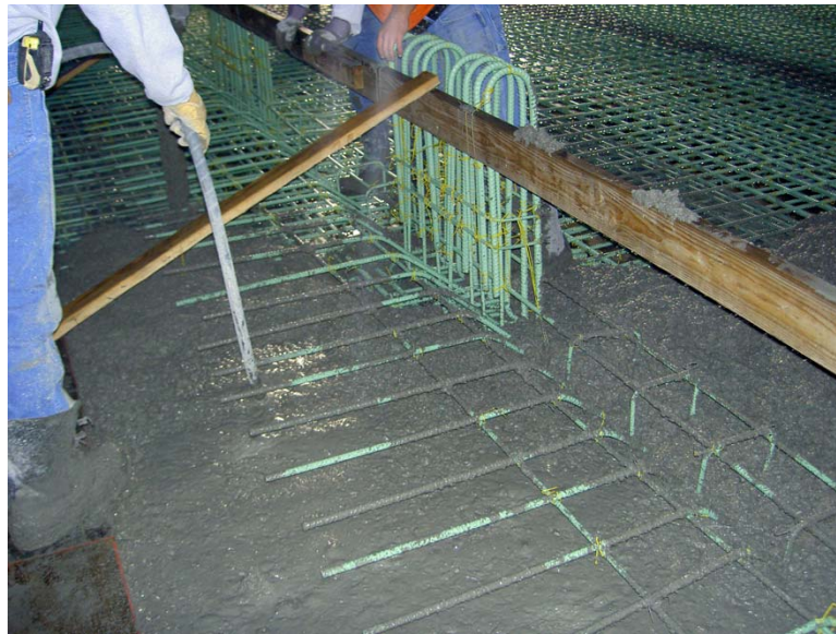
Fig. 5.9 Consolidation of the sidewalk portion of the deck
