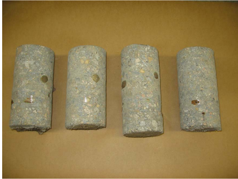
Fig. 5.17 – Cores from LC-HPC-10 qualification slab show coarse aggregate particles at or near the finished surface of the slab.
