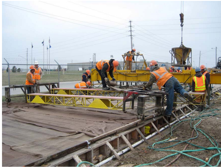
(a) Burlap rolled out onto the work bridge
