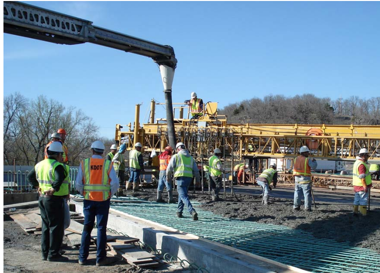
(c) For the south portion of deck the drop was approximately 4.6 m (15 ft)
