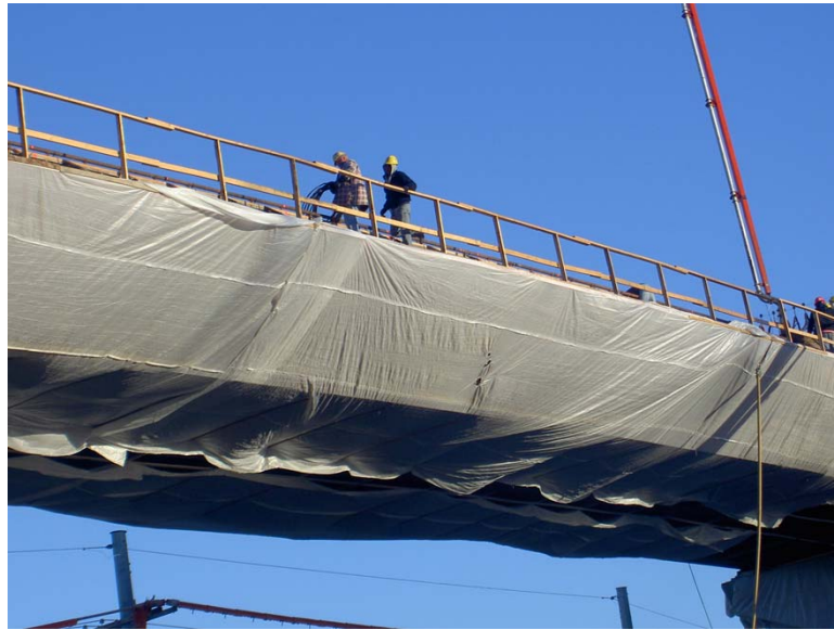
Fig. 5.31 Girders wrapped for cold weather curing requirements.
