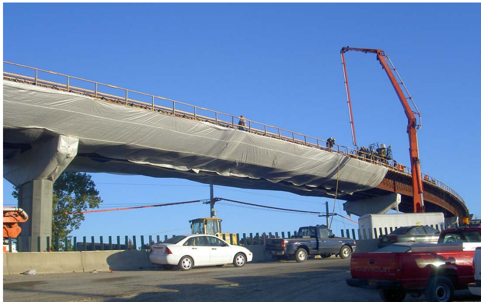
(b) Pier #5 to just west of Pier #6
