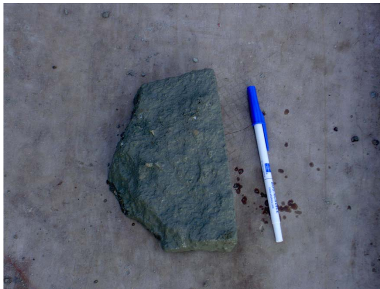
Fig. 5.27 A large coarse aggregate particle found in the concrete during the placement of LC-HPC-11
