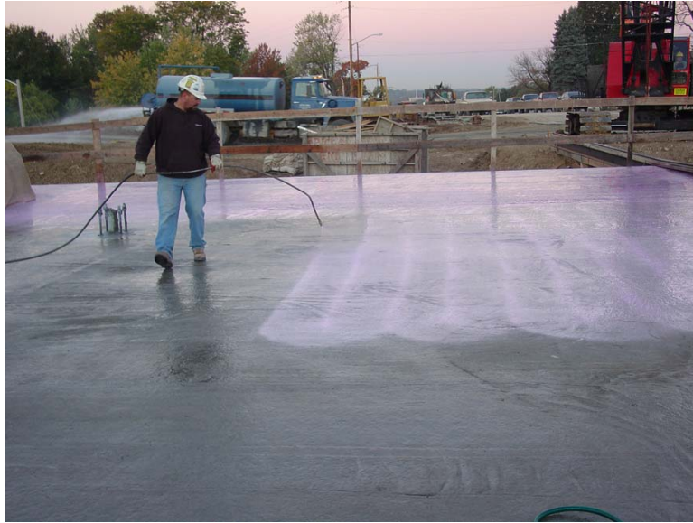
Fig. 5.4 (a) Application of the first coat
