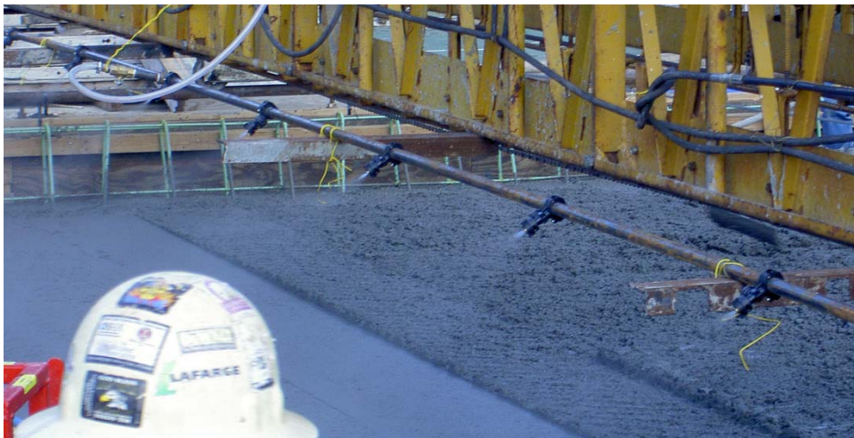
Fig. 5.29 Fogging equipment pointed down and spraying the concrete surface with water.
