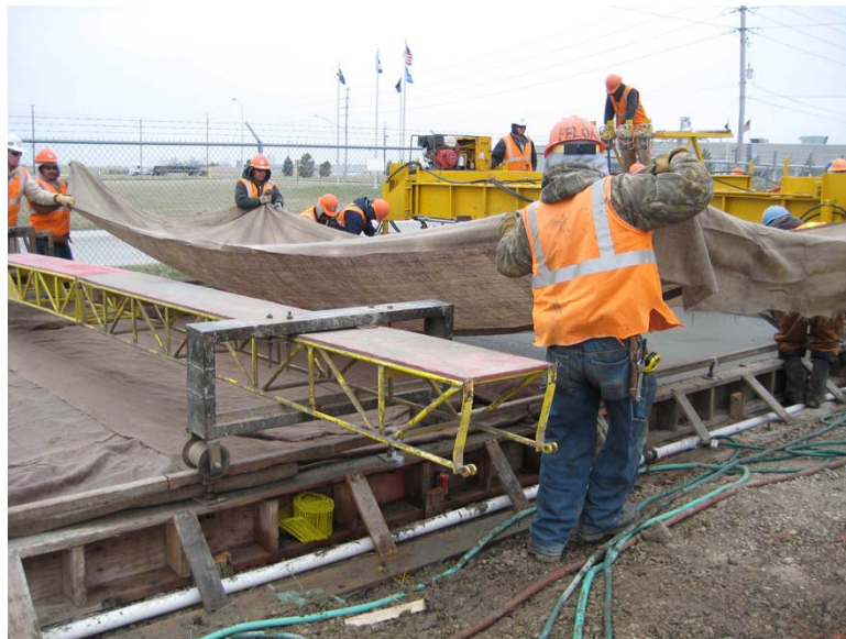
(b) Burlap placed from the sides of the deck
