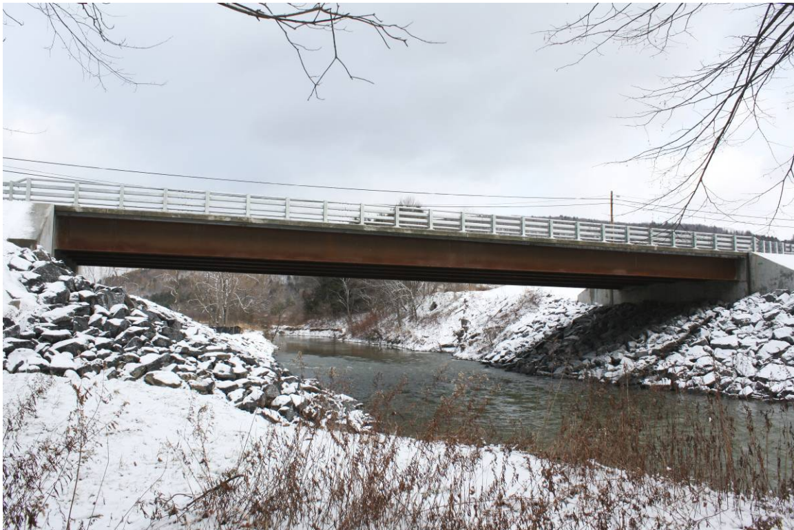
Figure 6. State Route 23 over Otego Creek near Oneonta, New York.
