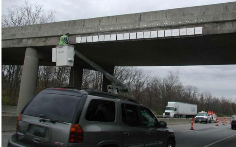
**Figure 12. Final installed I-Lam panel on bridge DEL-23-12.99 (Qiao P. , Yang, Mosallam, & Song, 2008).**
