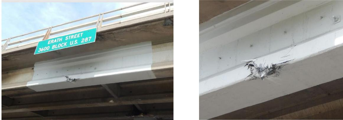
*Figure 32. Bridge beam hit with BPBW installed (Smith, 2014).*
