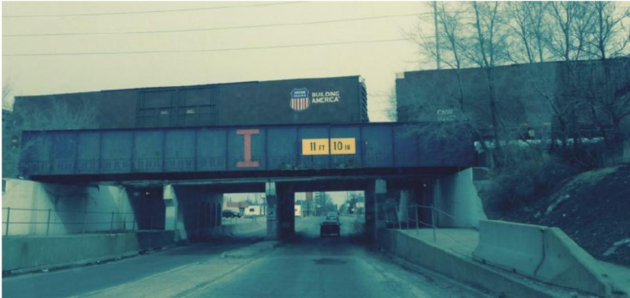
Figure 19. Typical through plate girder railroad bridge over a highway overpass (Xu, et al., 2022).
