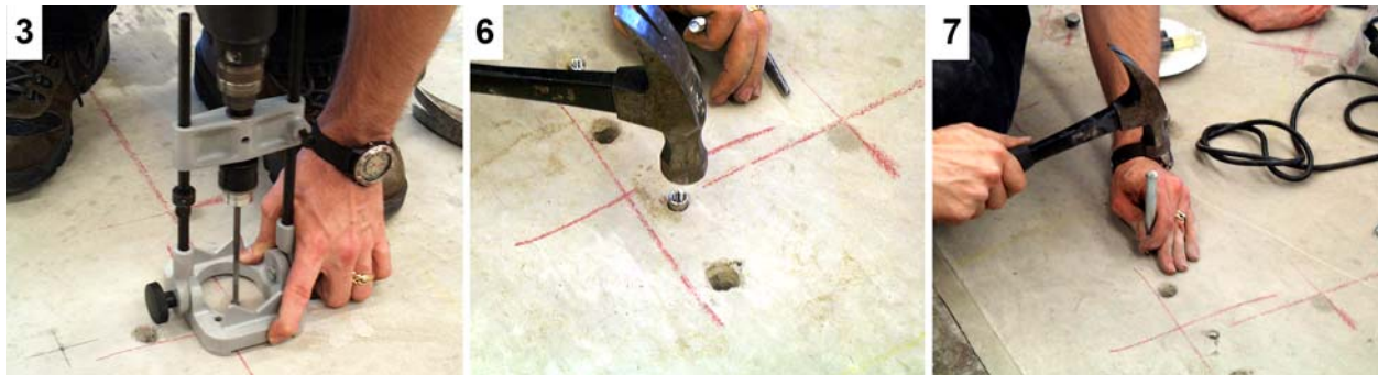
Figure 102. Photo. Concrete anchor installation, steps 3, 6, and 7.
