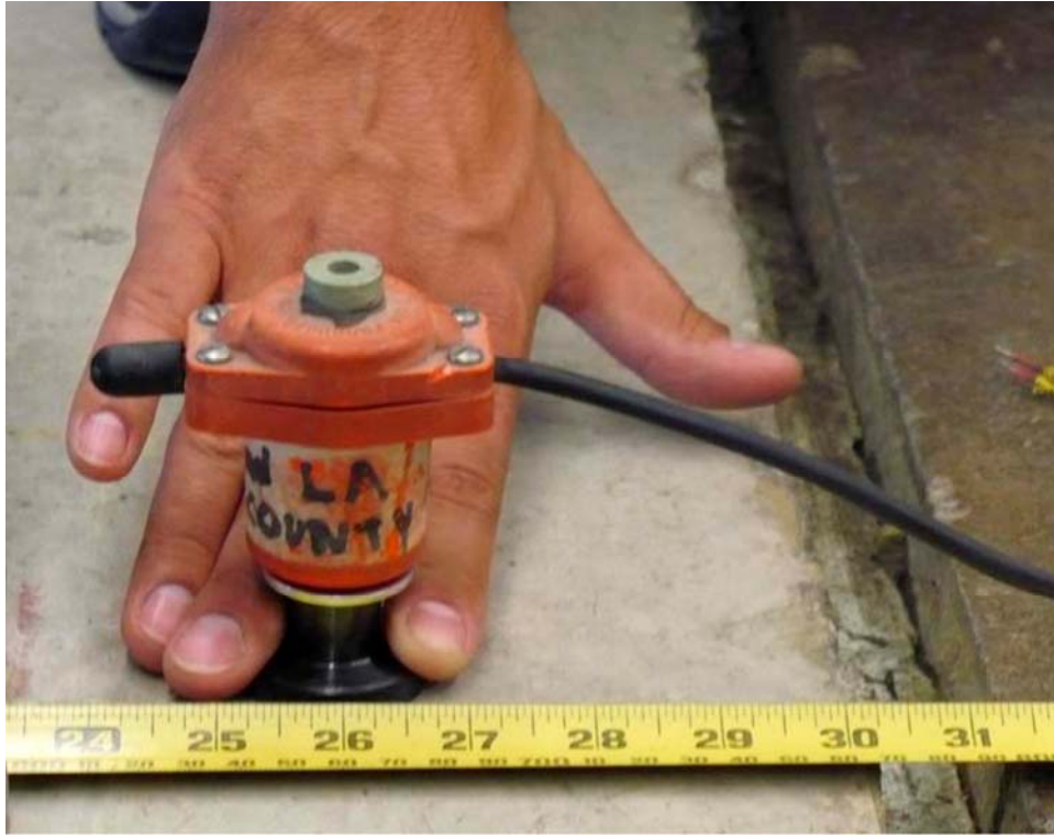
Figure 36. Photo. Locating a place to install the ball-joint floor anchor.
