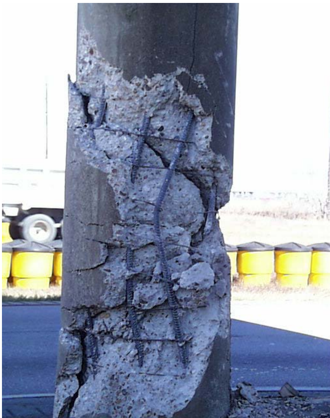
Figure 6 – Typical Failure Mechanism in Bridge Pier From Large Truck Collision.
