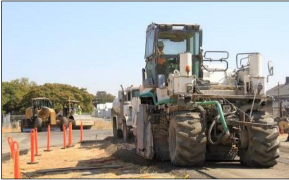
Figure 307. Photo. Test track recycling - 1.
