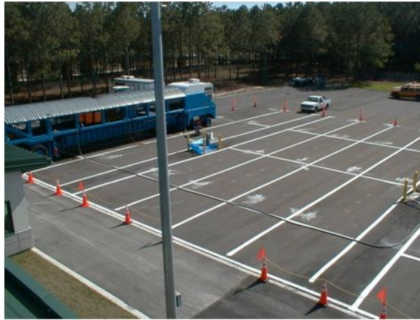
Figure 283. Photo. HVS test tracks.
