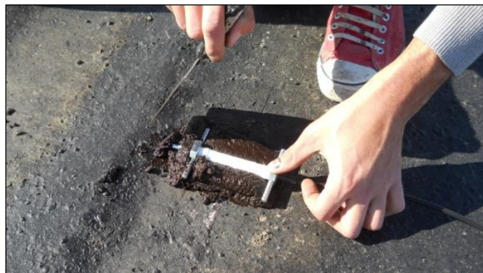
Figure 321. Photo. Installation of Tokyo Sokki KM100-HAS strain gauge.
