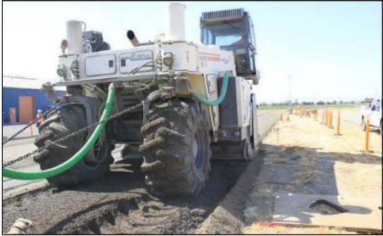
Figure 308. Photo. Test track recycling - 2.
