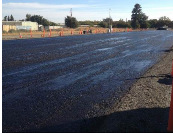
Figure 310. Photo. Primed surface.
