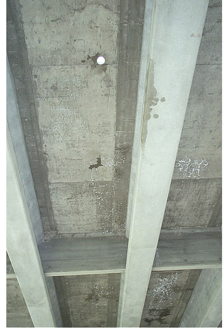
Figure 7. Photographs of core site (left) and from beneath bridge deck (right) after coring operation. Hole from core T-2 is visible. Dampness permeating through cracks visible beneath the area of core T-1. White efflorescence common directly below regions covered with cold patch material.
