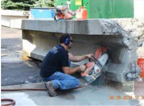
Figure 6.3-17 Cutting through the web with a circular concrete saw
