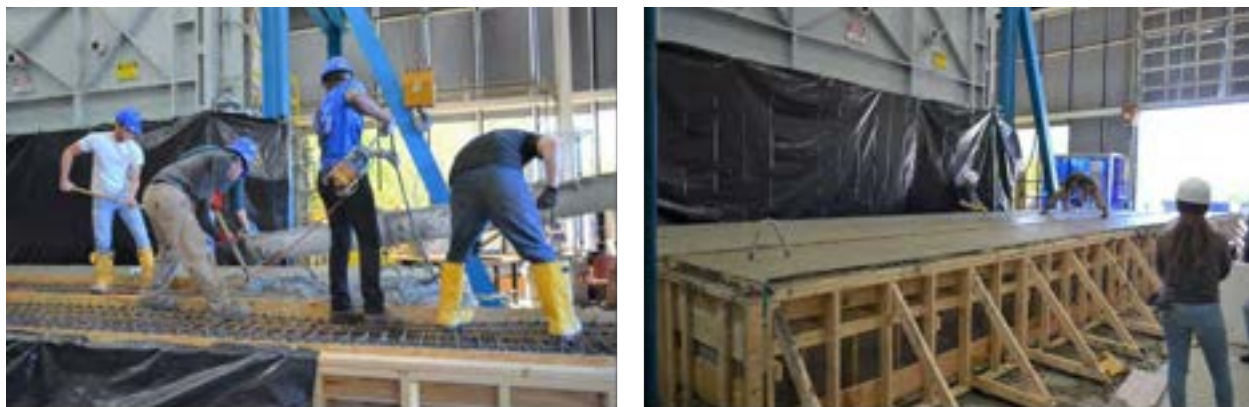
Figure 5.3-10 Casting concrete and finishing concrete surface for deck slabs
