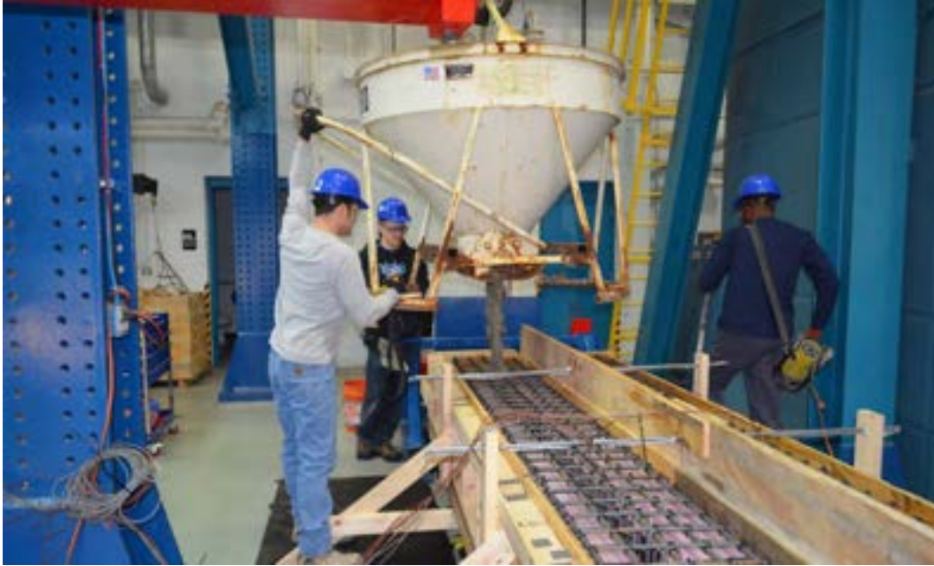
Figure 7.3-8 Pouring and compacting concrete
