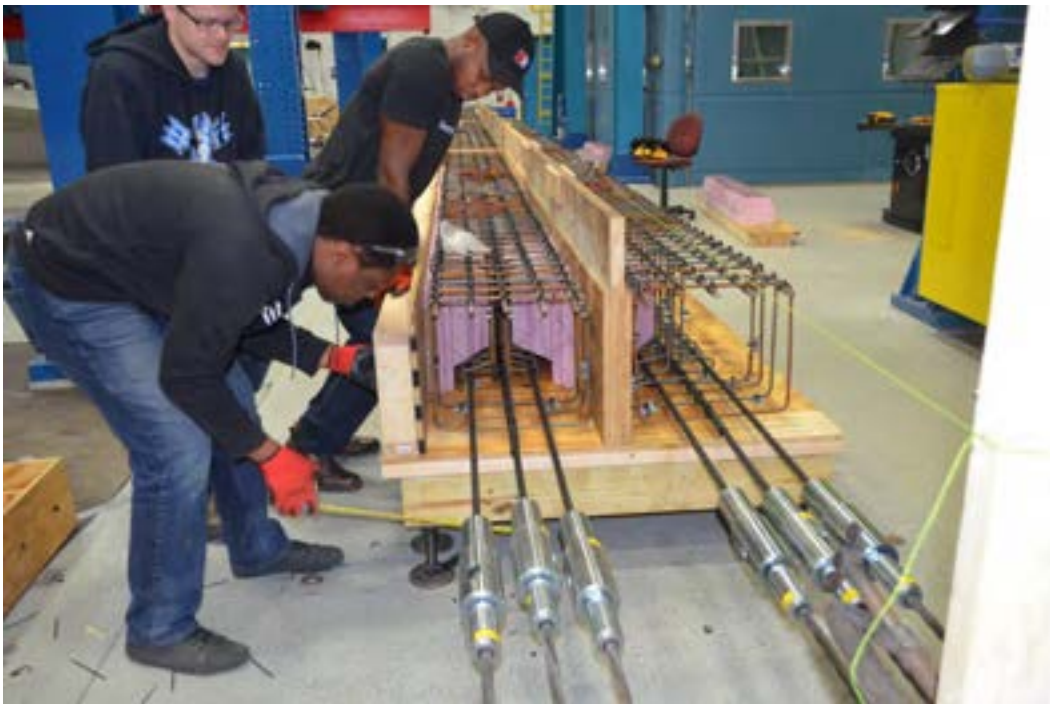
Figure 7.3-5 Coupler system for strand prestressing
