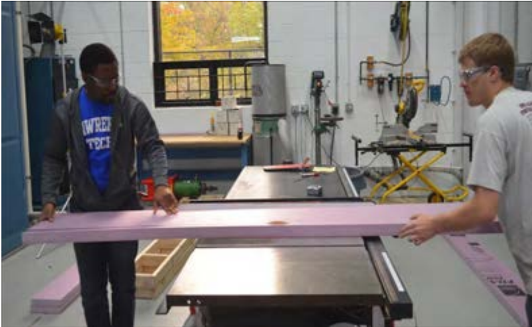
Figure 7.3-2 Preparing and cutting the formwork for the beams
