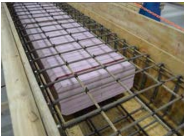
Figure 6.3-7 Assembling the reinforcement cage around the molded Styrofoam
