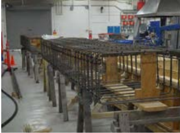
Figure 6.3-8 Tying and placement of reinforcement cage on prestressing bed
