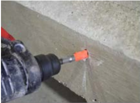
Figure 6.3-23 Installation of thermocouple into AASHTO I-beams
