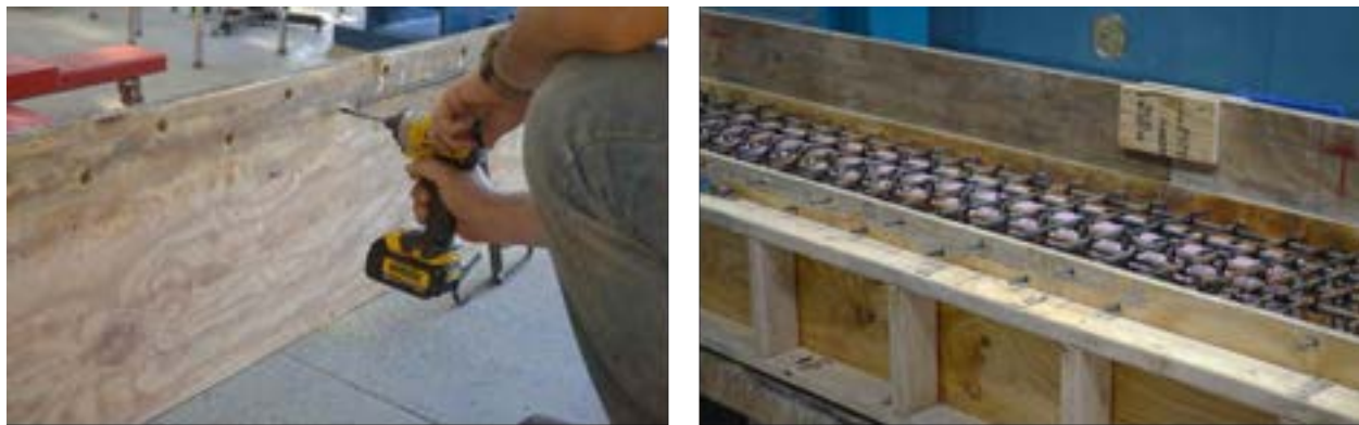
Figure 8.5-4 Drilling holes in the side walls of the formwork to accommodate for the pultrusion of the T-shape stirrups at the top flange of the beams
