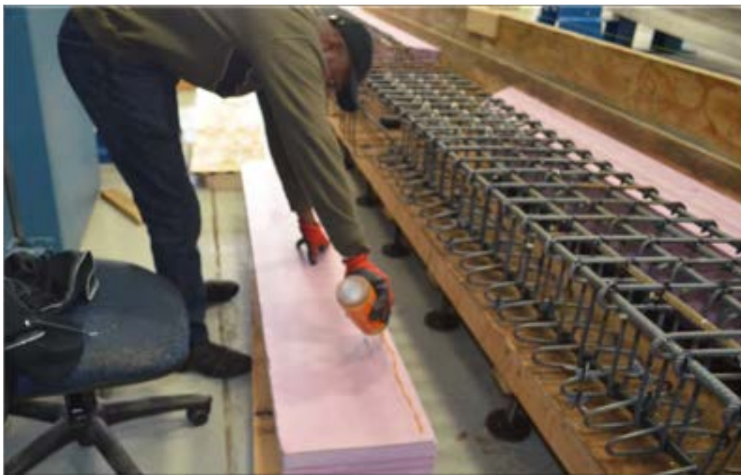
Figure 7.3-3 Building the sides of the formwork
