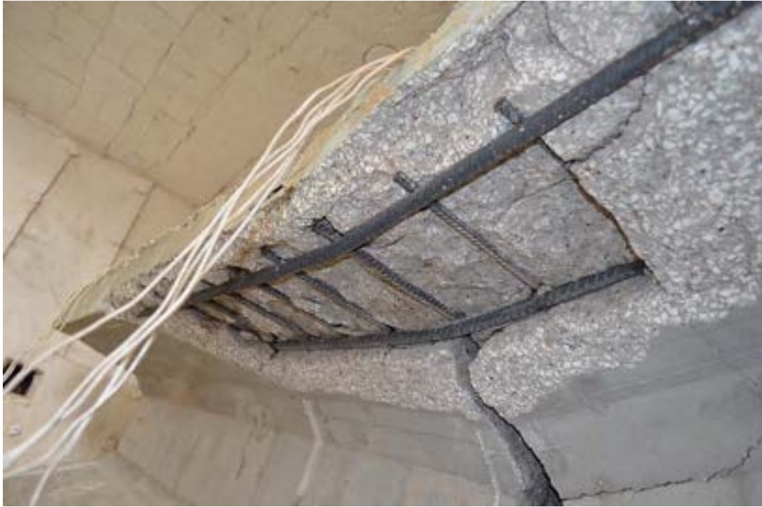
Figure 6.3-47 Spalling of concrete at top flange of beam
