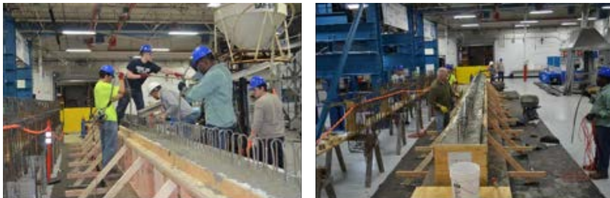
Figure 5.3-3 Concrete casting of AASHTO I beams
