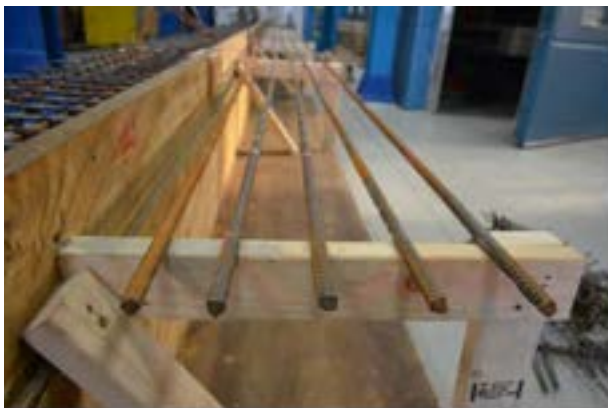
Figure 8.4-2 Assemblage of the reinforcement cage from steel rebars and steel stirrups
