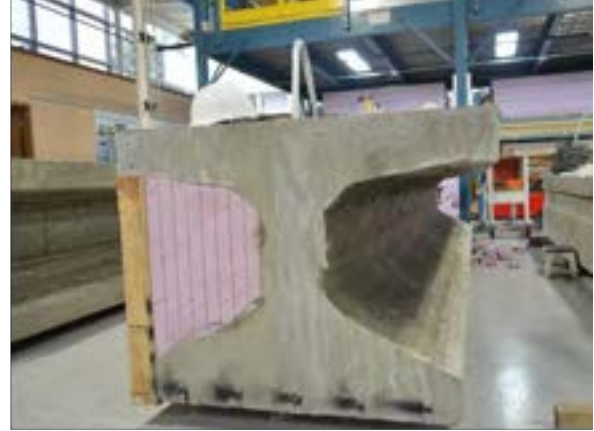
Figure 6.3-14 Removing the formwork of the beams
