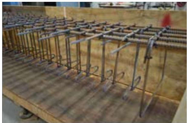
Figure 8.4-2 Assemblage of the reinforcement cage from steel rebars and steel stirrups
