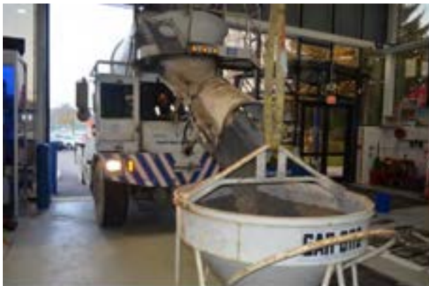
Figure 8.4-6 Placing concrete into the formwork and compacting using electric pencil vibrators
