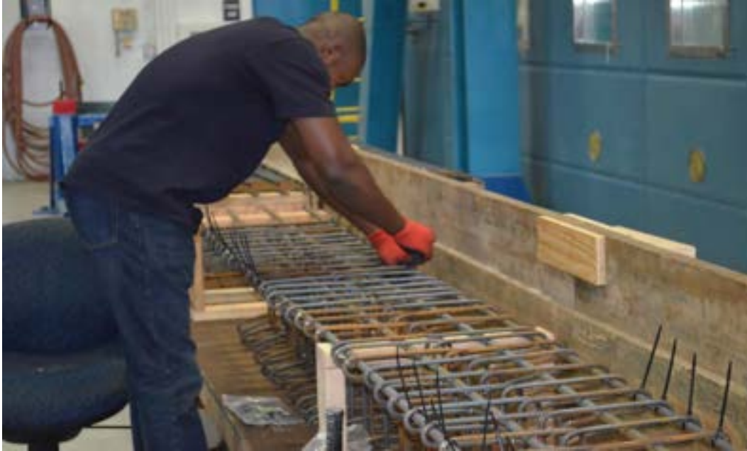
Figure 7.3-4 Assembling reinforcement cages from steel stirrups and top steel reinforcement
