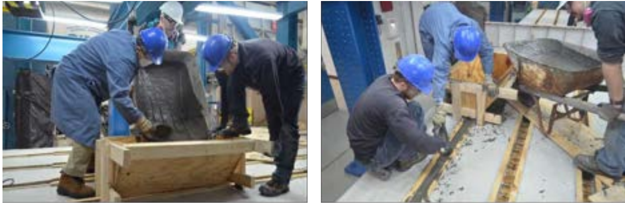
Figure 8.5-11 Pouring UHPC into shear key joints
