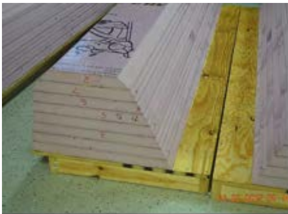
Figure 6.3-6 Attachment of Styrofoam to side walls of the form
