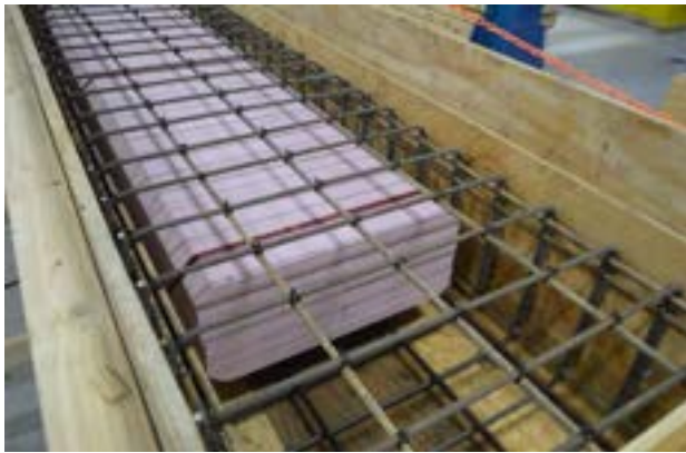
(c) Reinforcement cage of box beam section
