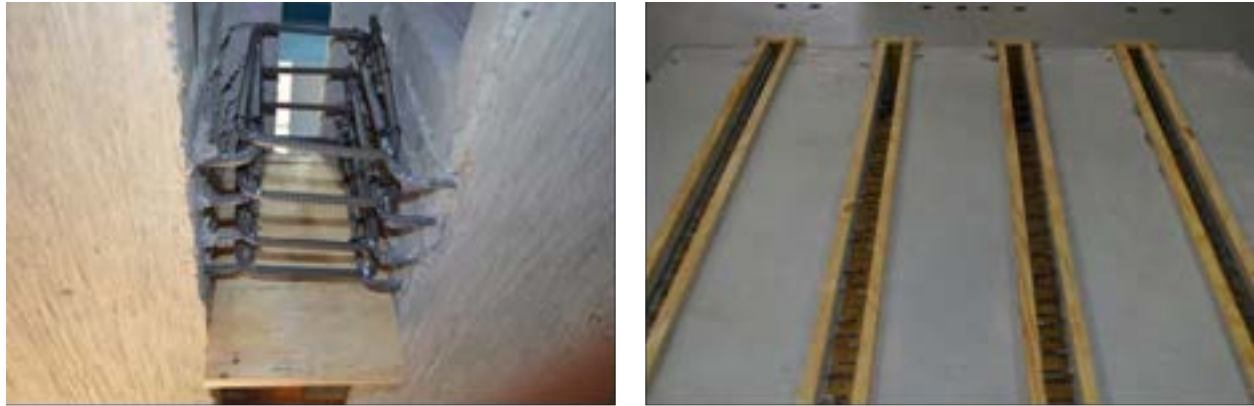
Figure 8.5-8 Formwork and reinforcement configuration for shear key joints
