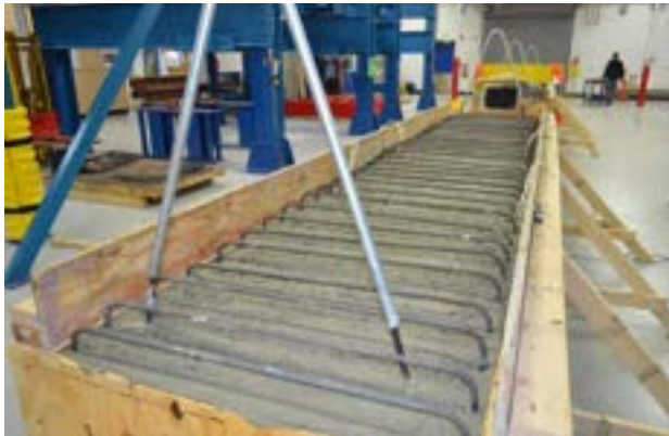
(e) placing concrete in box beam formwork
