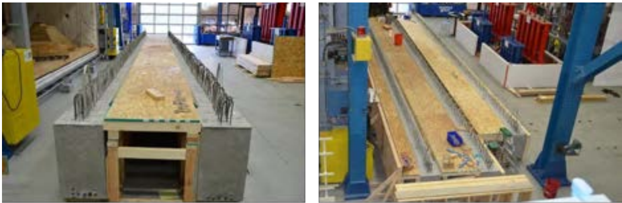
Figure 5.3-8 Building formwork for the deck slab of AASHTO I-beams
