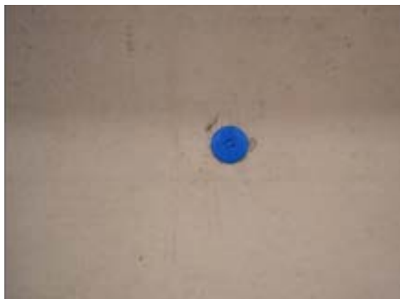
Figure 6.3-20 Installation of the sleeve and the RH Probe sensor
