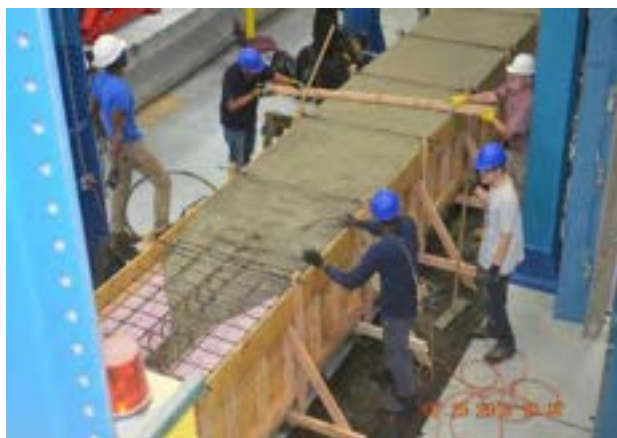
(c) Placing concrete inside formwork
