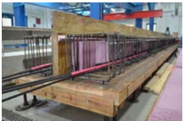
Figure 8.4-3 Passing prestressing CFCC strands inside the reinforcement cage and shielding the debonded strands from concrete using polyethylene pipes
