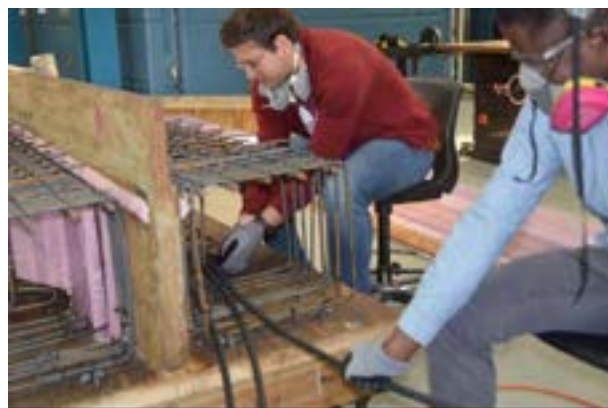
Figure 8.4-3 Passing prestressing CFCC strands inside the reinforcement cage and shielding the debonded strands from concrete using polyethylene pipes
