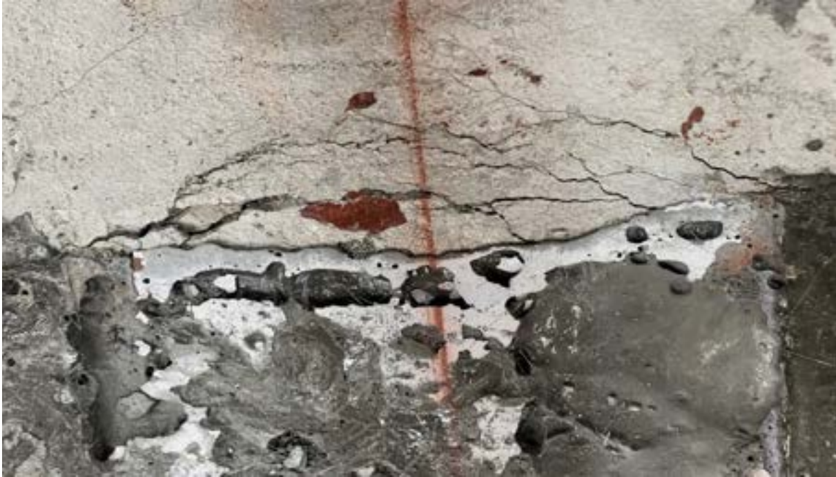
Figure 8.8-12 Surface cracks at the concrete side of shear key joints
