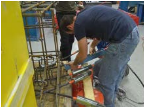
Figure 6.3-9 Installation of prestressing anchorage and prestressing of strand
