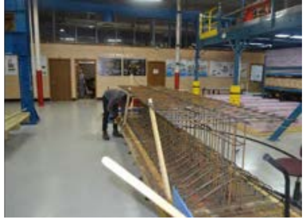
Figure 6.3-8 Tying and placement of reinforcement cage on prestressing bed
