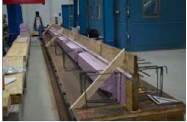
Figure 8.4-1 Setting up the wooden center walls and attaching the Styrofoam to center walls
