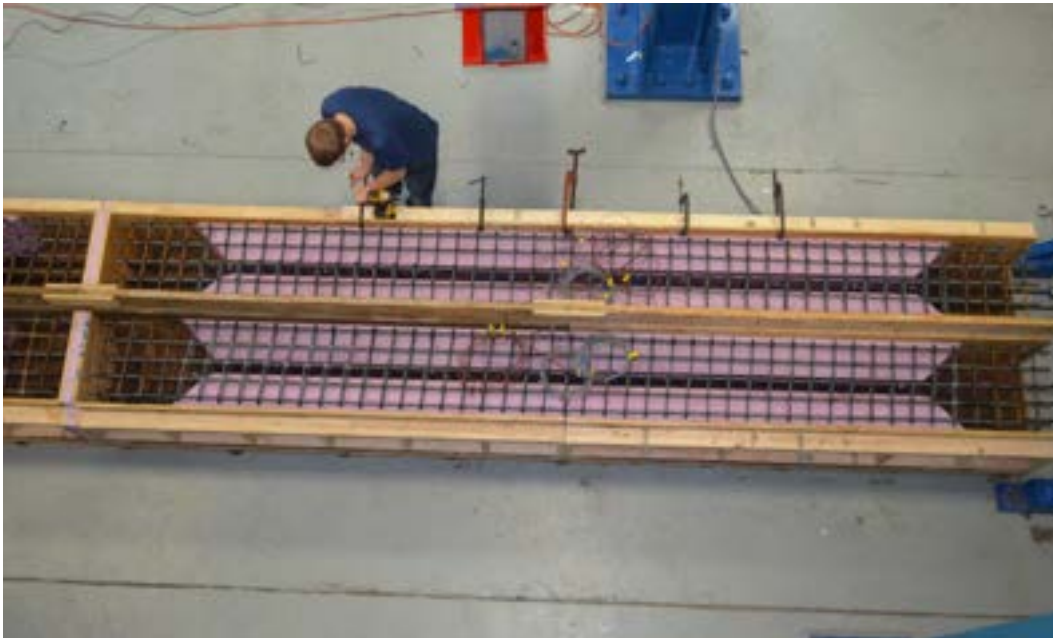
Figure 7.3-7 Completing the formwork
