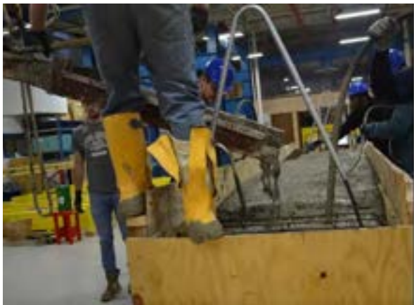
Figure 6.3-10 Concrete casting
