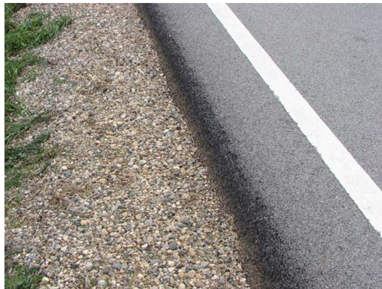
Figure 3. Exposed Safety Edge
