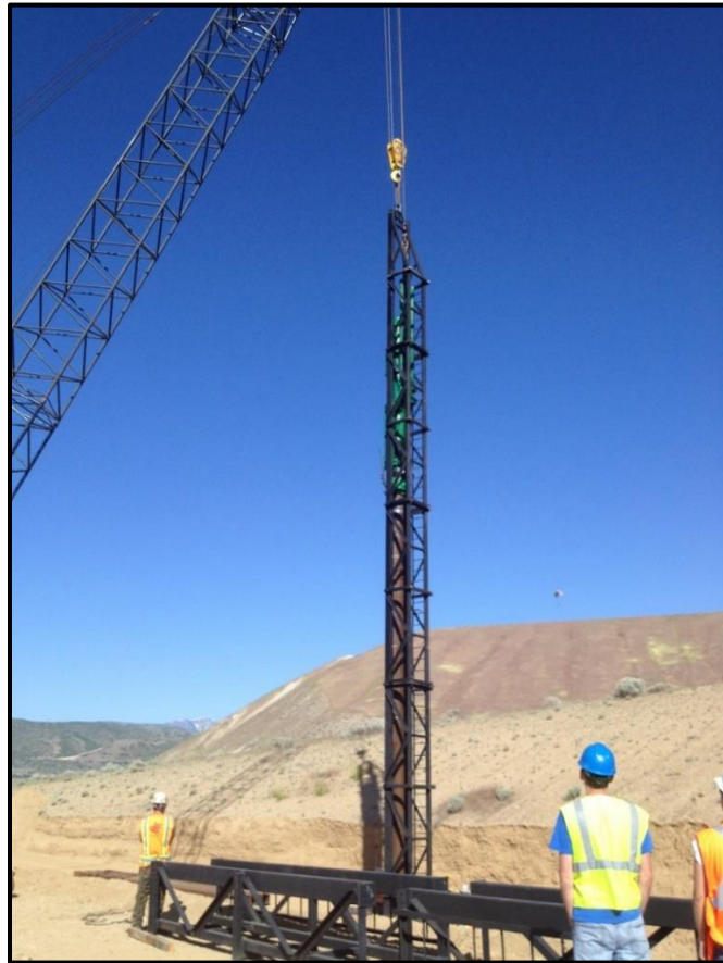
Figure 3-3: Installation of piles using a diesel hammer.
