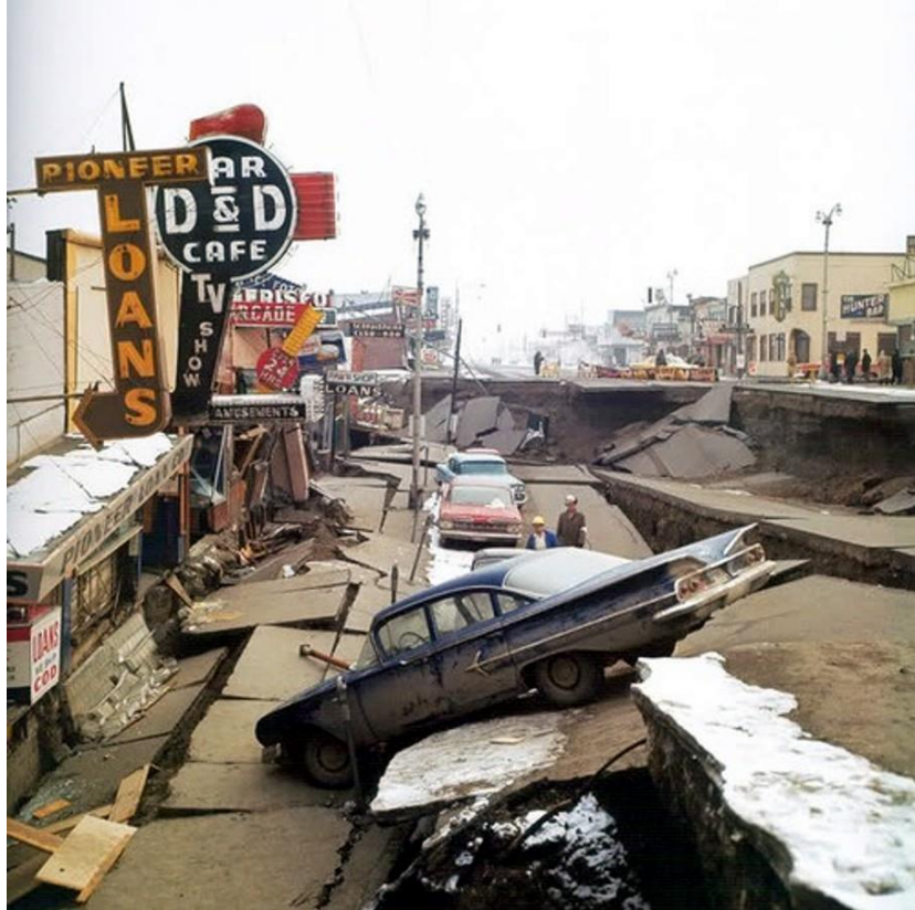
Figure 1-2 Downtown Anchorage, AK Experienced Flow Deformation and Lateral Spreading Which Caused Downhill Slumping Towards the Harbor as a Result of Liquefaction Caused by M_w 9.2 Earthquake of 1964.
