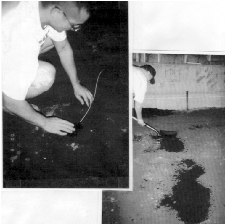
Figure 2.5.3.2: Strain gage being installed prior to paving.
