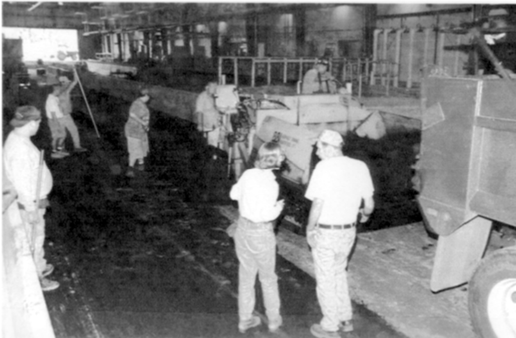
Figure 2.1.2: FERF with test sections under construction.
