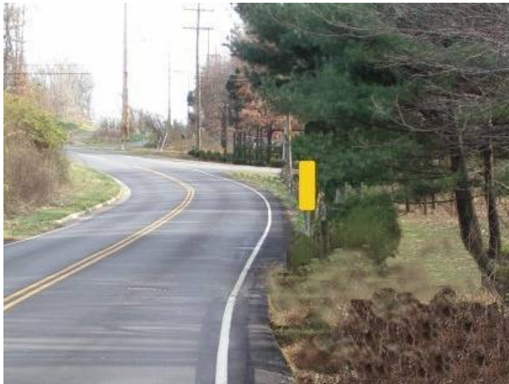
Figure 3: Example of an Object Marker Alternative as Shown in the Comprehension Survey.
