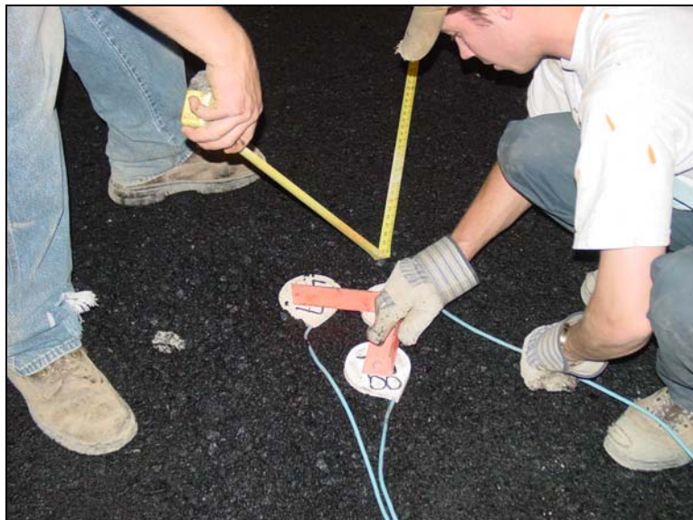
Figure 22. Installing \epsilon mu coils in the hot asphalt concrete.
