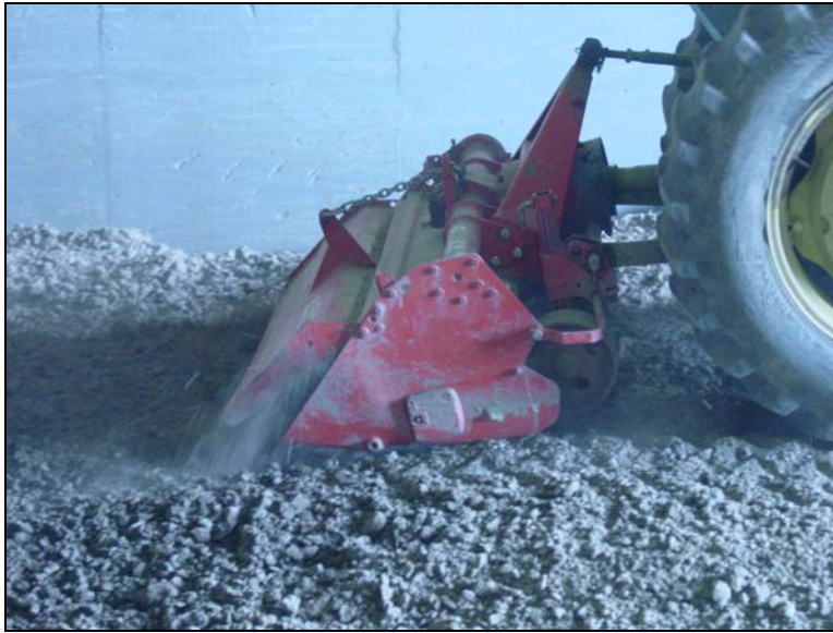
Figure 15. Cultivating the soil to facilitate moisture absorption and uniform distribution.
