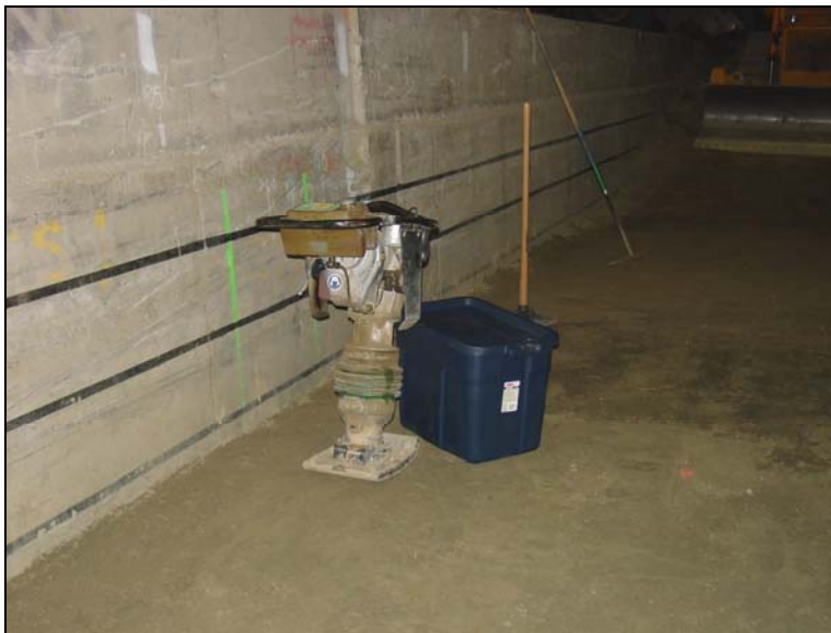
Figure 16. Plate compactor used to compact the edges of the test section.
