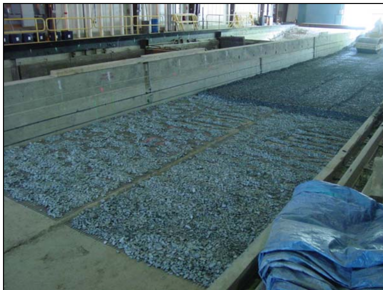
Figure 24. Geogrid partially covered with base course aggregate.
