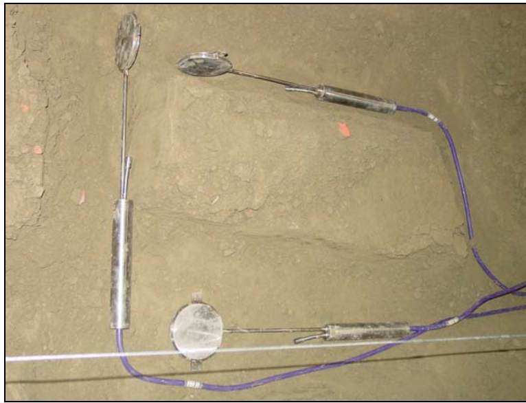
Figure 20. Top view of pressure cells during installation, showing trenches and cable.
