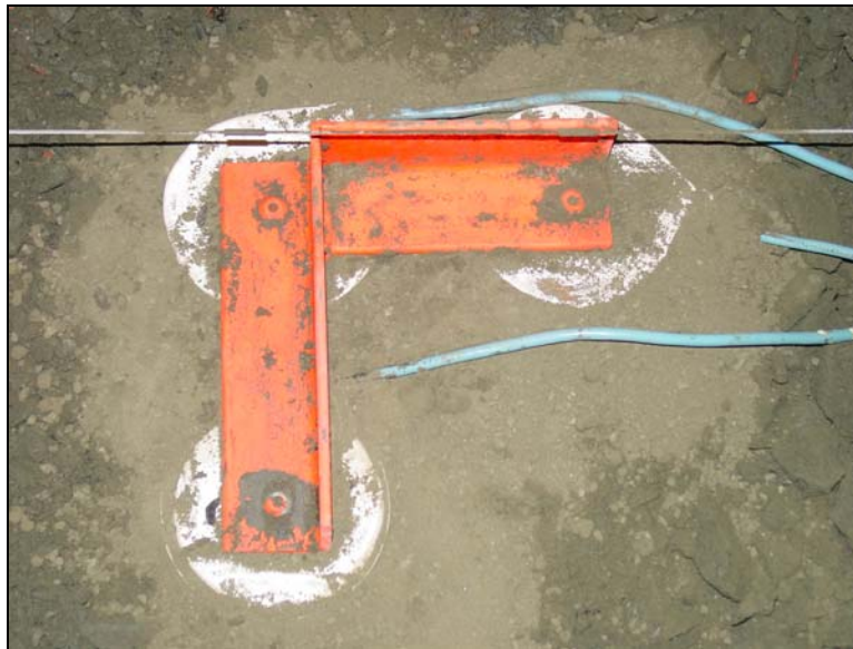
Figure 21. Installation mold for placement of three \epsilon mu coils.
