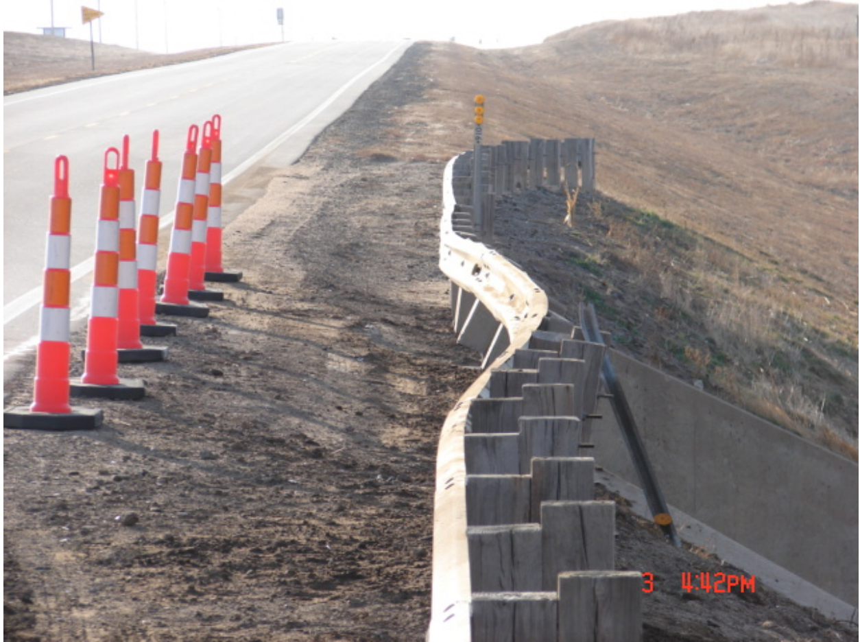
Figure 5. Guardrail Adjacent to Culvert
