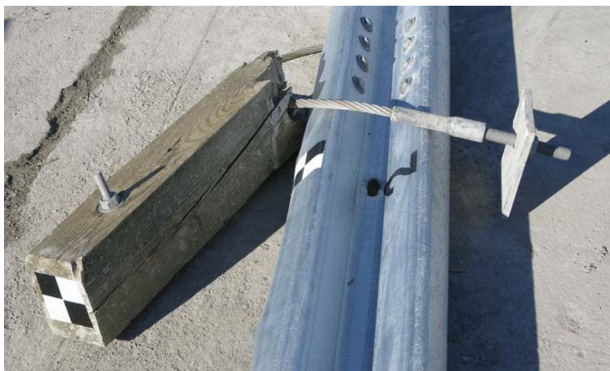
Figure 5. Damage to Upstream Anchorage System - Test MWTSP-1
