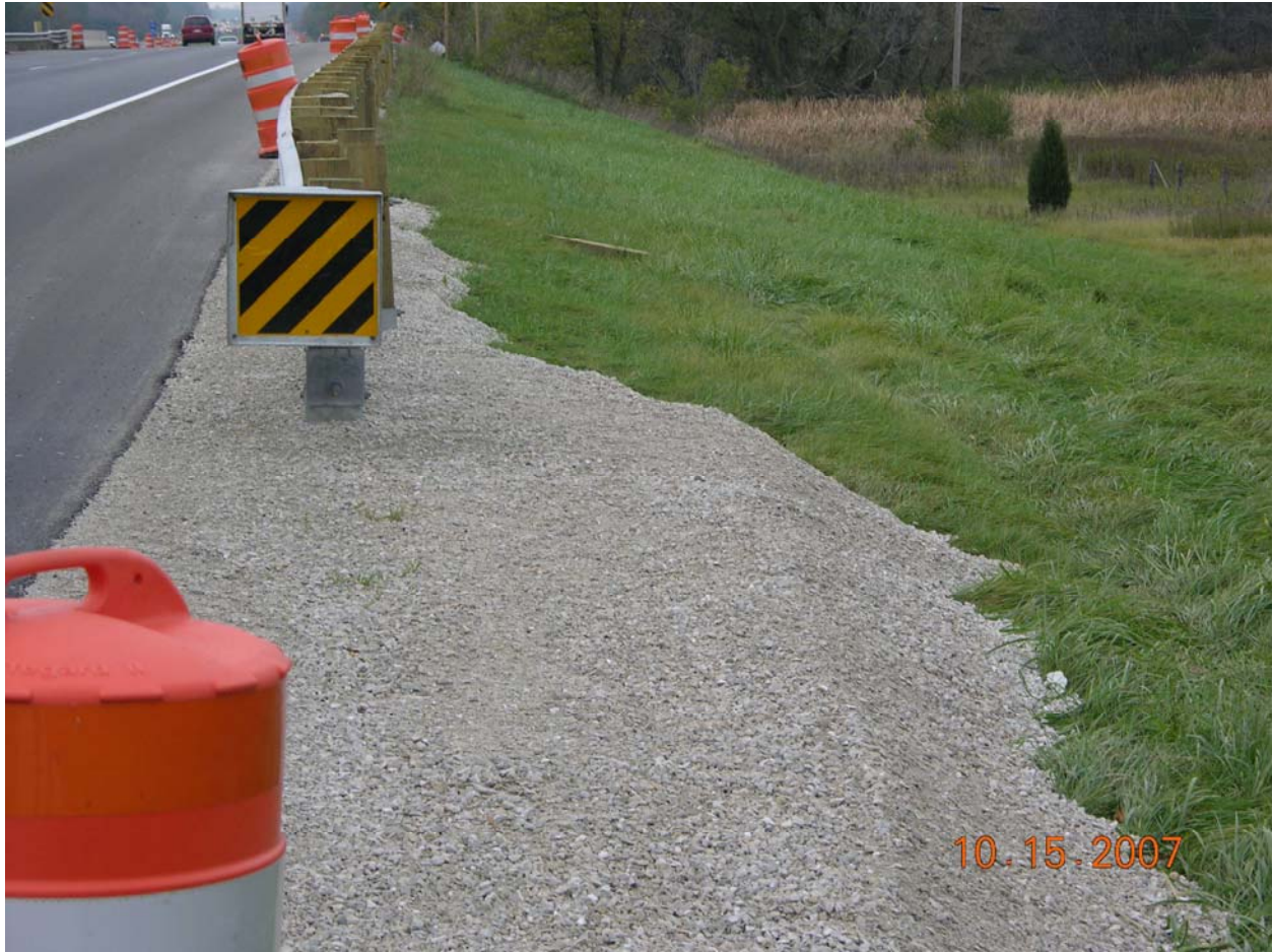
Figure 1. End Terminal Slope
