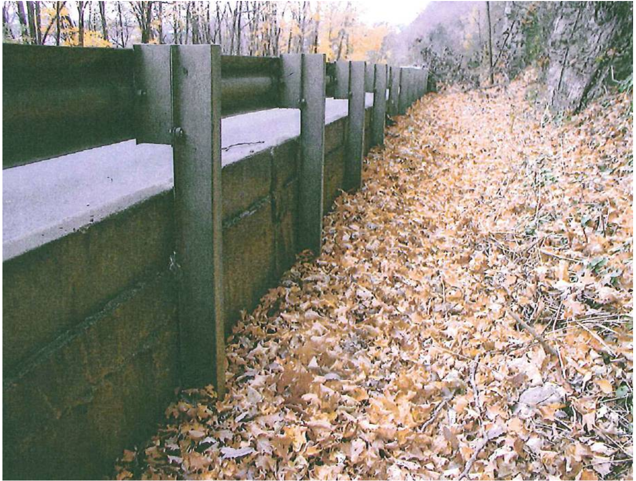
Figure 4. Guardrail Adjacent to Retaining Wall
