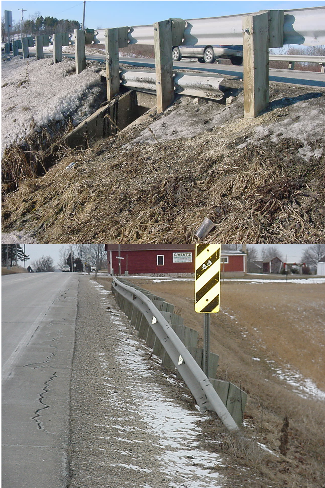
Figure 9. Guardrail on Slope Installation
