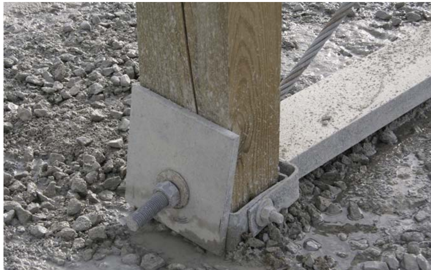
Figure 4. Upstream Anchorage System - Test MWTSP-1
