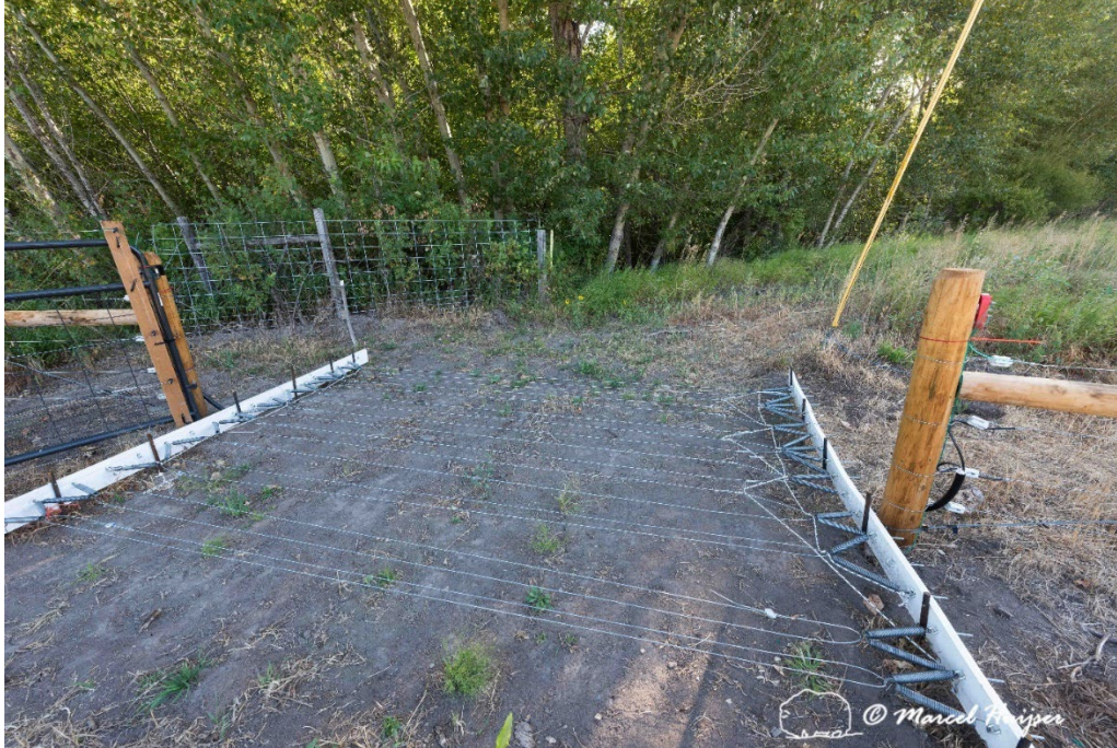
Figure 8: The drive-over wires, about 14'3" (4.34 m) wide (post-post) and 10'2" (3.10 m) long. The 18 drive-over wires are about 7" (18 cm) above the ground and the gaps between the wires vary between 5-12" (13-30 cm). There are "side-board" wires that angle toward the ground from the post along the sides of the barrier to reduce the likelihood of an animal bypassing the drive-over wires. However, these "side-boards" do not cover the full length of the barrier.
