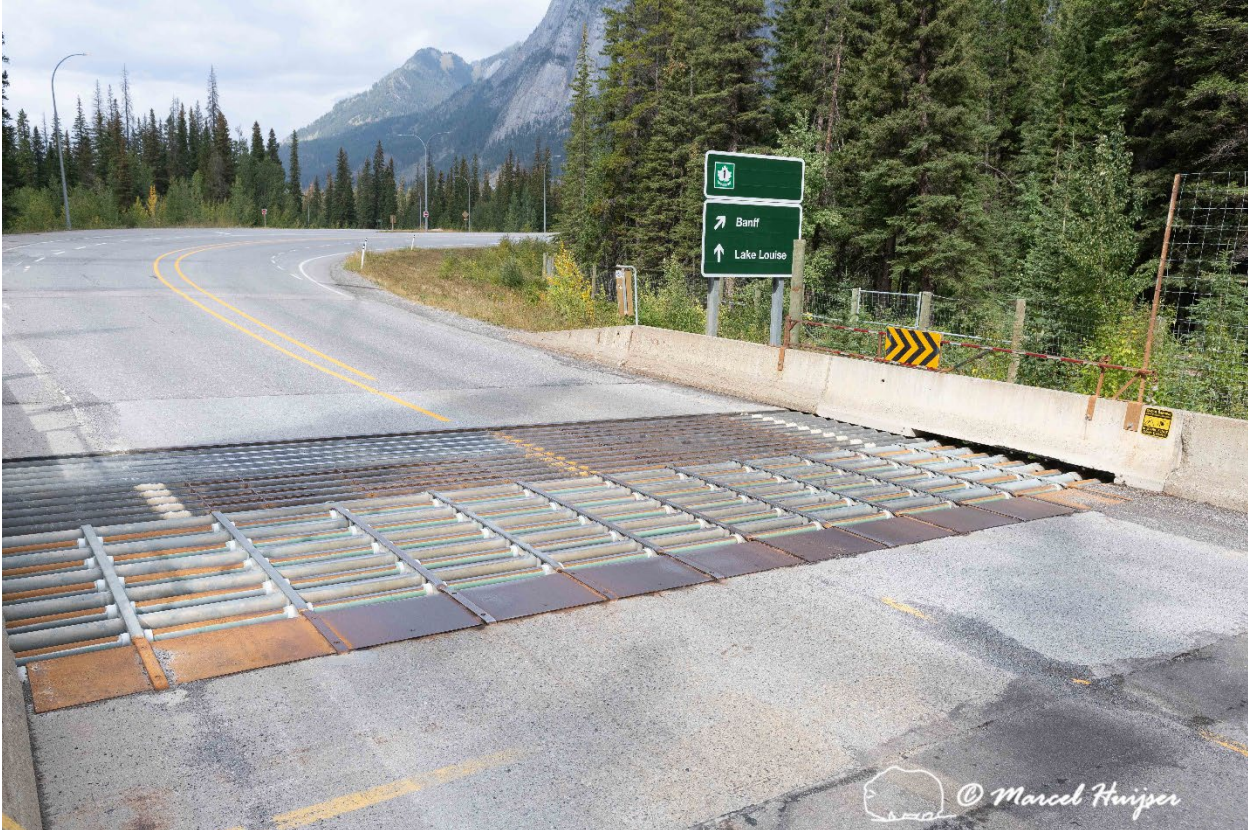
Figure 26: Electrified barrier, Sunshine Road, Banff National Park, Canada.
