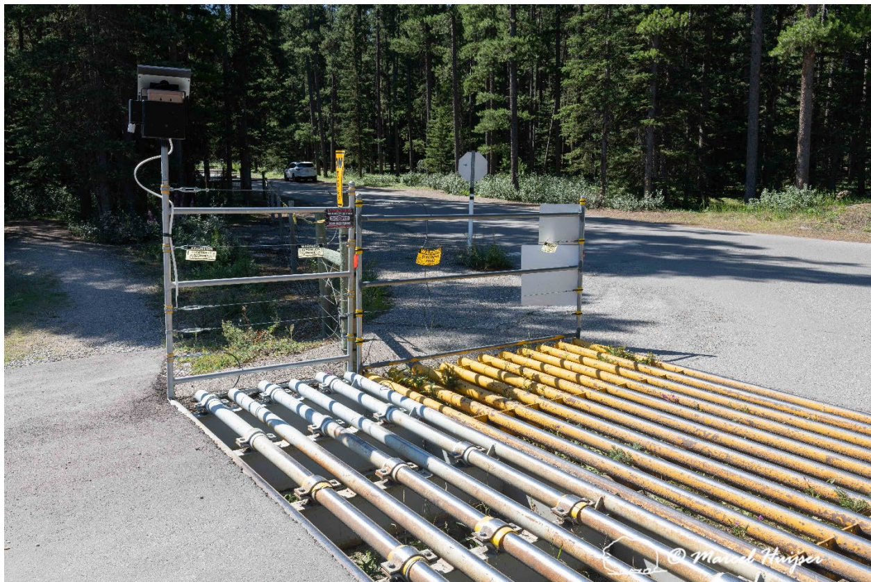
Figure 28: Electrified barrier, Lake Louise Campground, Lake Louise, Canada.
