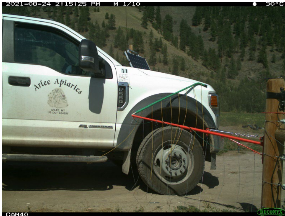
Figure 23: Broken horizontal pole of a bump gate because of a vehicle passing through.
