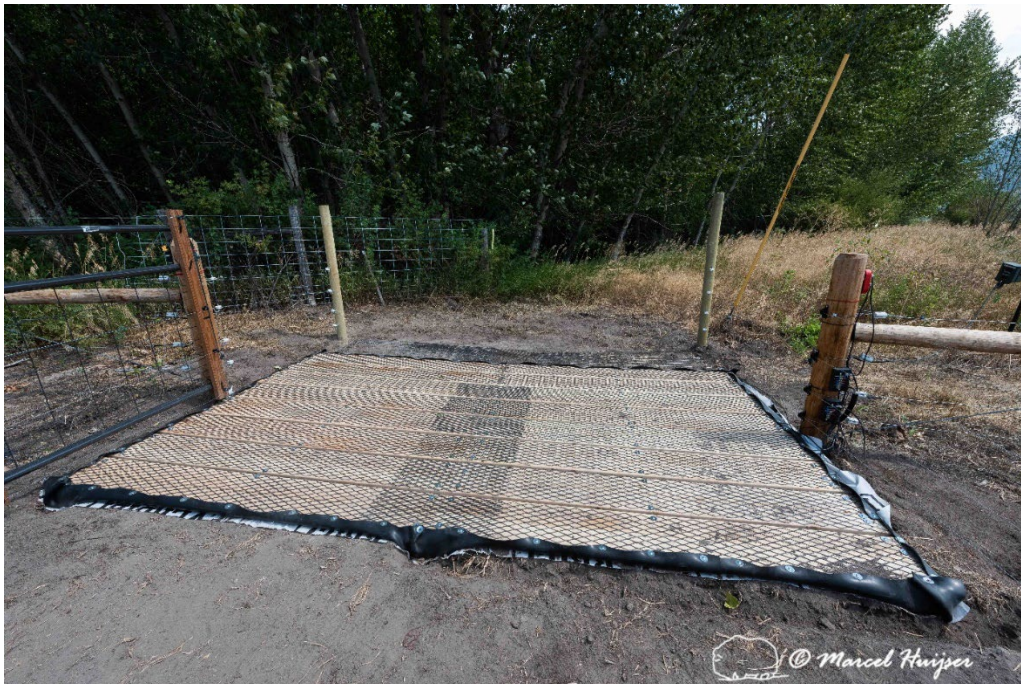
Figure 9: The drive-over mat about 14'3" (4.34 m) wide (post-post) and about 10' (3.05 m) long. On the far side, the habitat side, there is metal mesh on the ground, connected to a grounding rod (about 2 ft (61 cm) wide). This is followed by 8 sections of 10-11" (25-28 cm) wide expanded metal sheeting (alternating positive and negative (ground)) mounted on wooden planks. This drive-over mat is powered by its own solar panel, battery and energizer.
