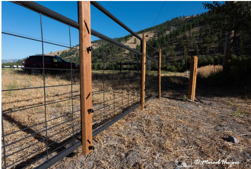
Figure 5: The electrified swing gate (16' (4.88 m) wide, 4'6" (1.37 m) tall, about 7" (18 cm) gap between ground and bottom of gate). The wires were mounted at 6" (15 cm), 1'7" (48 cm), 3'2" (97 cm), and 4'7" (140 cm) above the ground.
