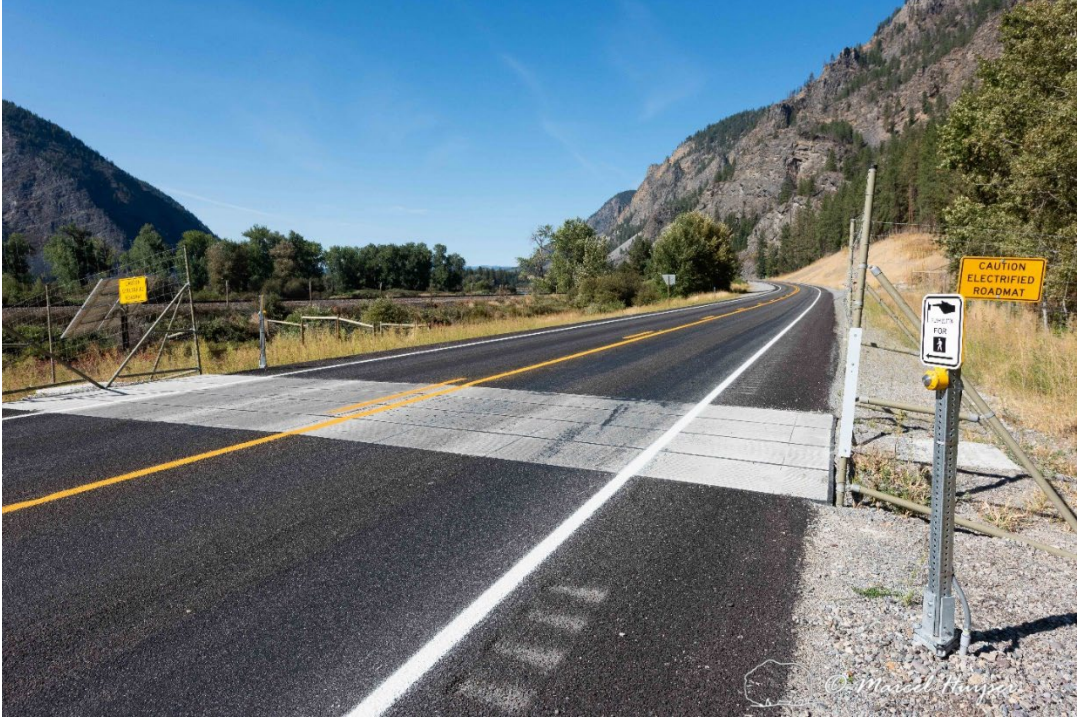
Figure 33: The electrified barrier at the east fence-end.
