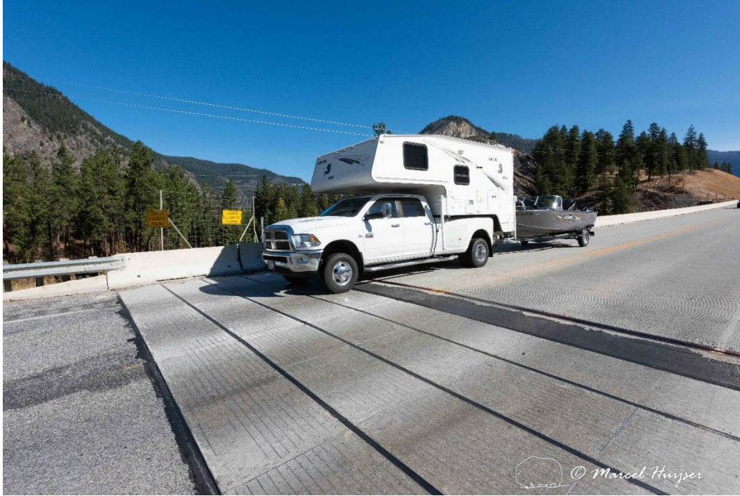
Figure 31: The electrified barrier at the west fence-end. Note that the bridge directly connects to the electrified barrier.
