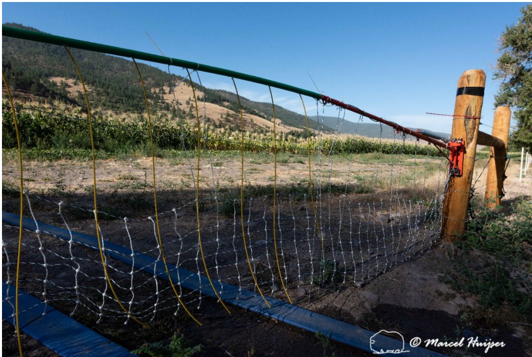
Figure 7: A modified drive-through bump gate (with conductive netting) (about 16' (4.88 m) wide, about 3' (91 cm) tall), with vertical electrified wires and custom conductive netting (about 2' (61 cm) high) attached.
