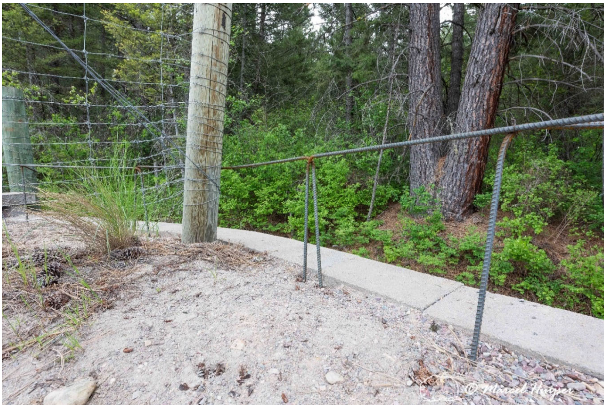
Figure 9: The legs of the “staples” and L-shaped corner elements were connected with metal wire.
