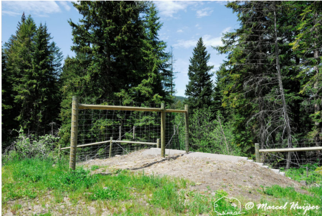
Figure 2: An unmodified jump-out in the Evaro area. The mount allows the animals to walk up to an opening in the fence, with a drop of around 6 ft (1.83 m) to the habitat side of the jump-out.
