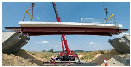
Figure 6: A hybrid traffic bridge over B3 highway in Germany (Fiberline Composites, 2006).
