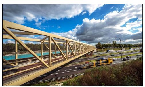
Figure 14: Hybrid bridge with FRP decking in Utrecht, the Netherlands (FiberCore Europe, 2012).
