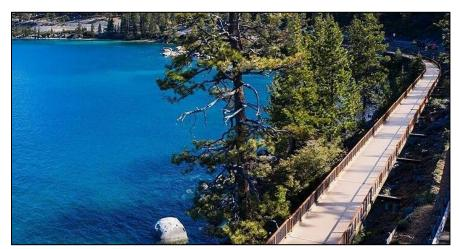
Figure 13: Hybrid walkway with FRP decking and steel supports near Lake Tahoe, California (Creative Composites Group, 2019).
