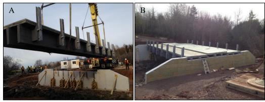
Figure 17: Wood and FRP bridge made by Guardian Bridge Rapid Construction for a two-lane road; A) a triple-tee span being placed by a crane; B) all three spans placed on top of an FRP abutment.
