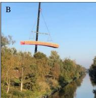
Figure 10: A) FRP uni-mold bridge is delivered in one piece from the factory to the construction site; B) bridge is installed using one crane (FiberCore Europe, 2019b).
