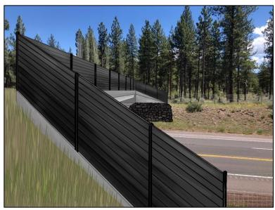
Figure 39: Recycled-plastic sound and light barrier installed on top of soil-retaining concrete curb.
