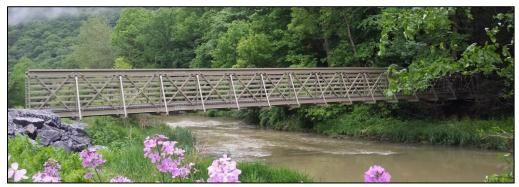
Figure 11: FRP Pultrusion pedestrian bridge built by Creative Pultrusions (Griffith, 2018).
