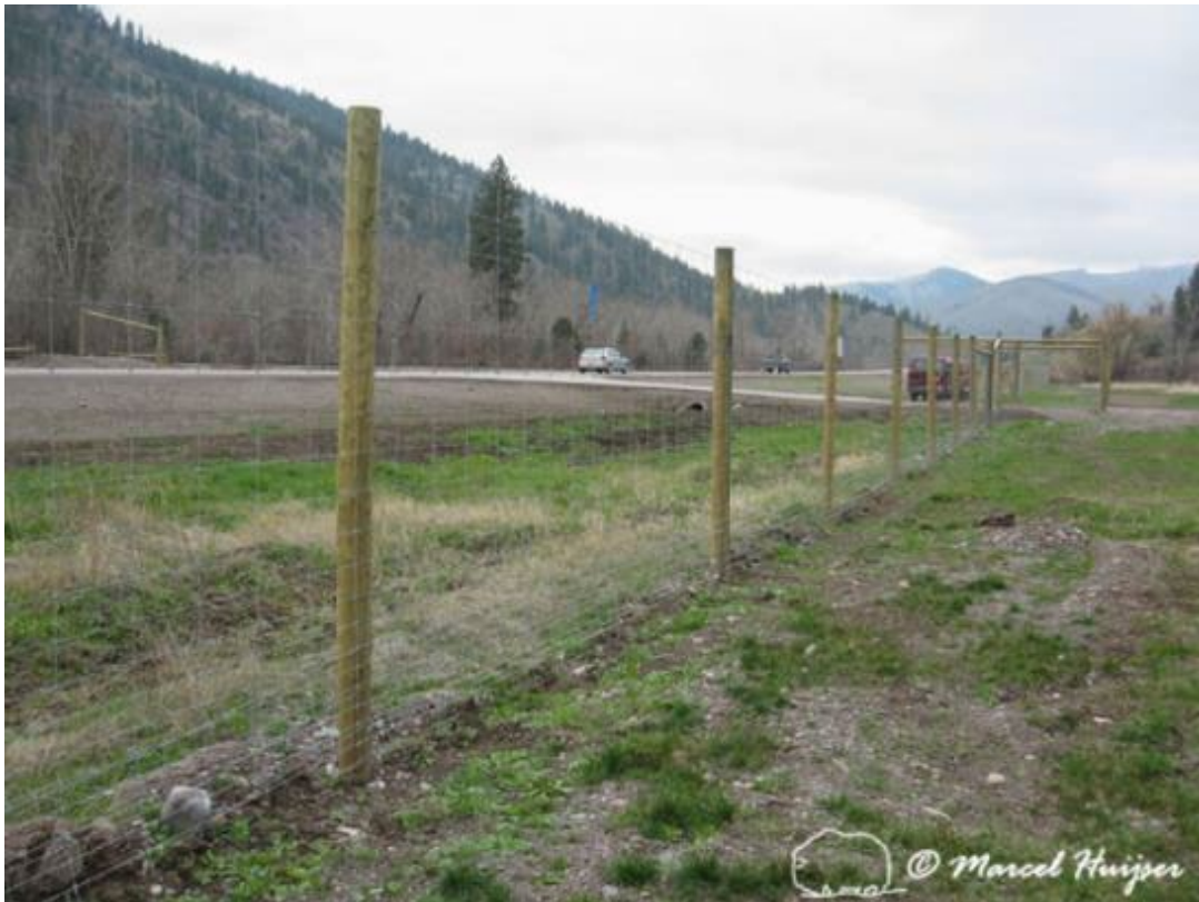
Figure 24. Typical large ungulate (hoofed animal) fence in North America, 8 ft tall, wooden posts and mesh-wire fence material, US Hwy 93 North, Montana, USA. Note that there is a dig barrier (e.g., for canids (dog family members)) attached to the main fence material at the bottom is buried in the ground.
