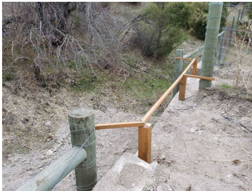
Figure 23. A jump-out that is modified with a 2 in (5 cm) by 2 in (5 cm) bar for the design experiment.
