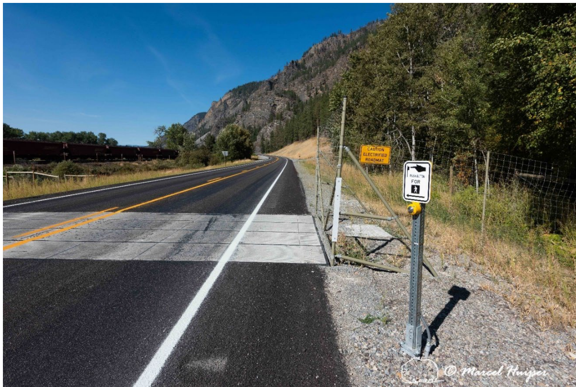
Figure 14. An example of an electrified barrier at a fence-end.
