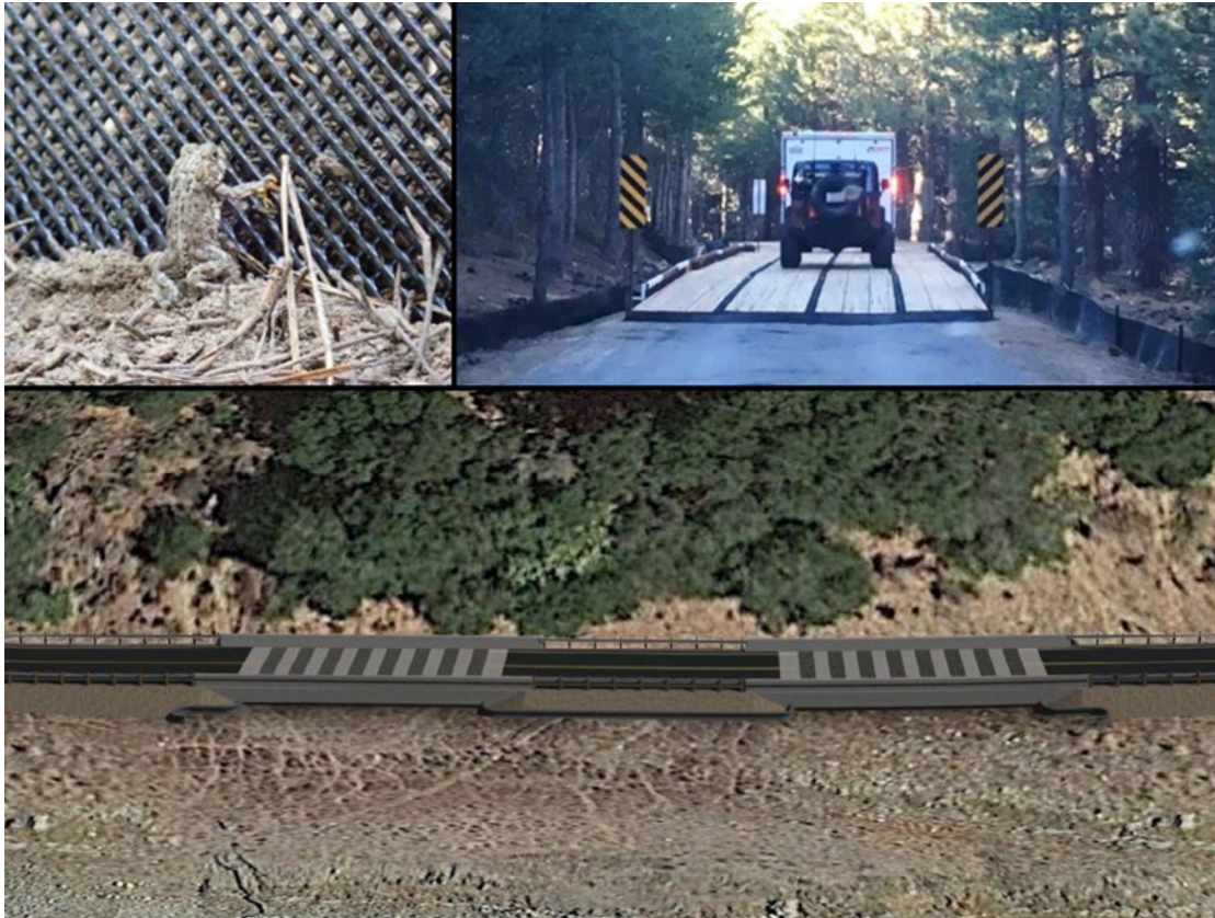
Figure 20. Elevated Road Segment (ERS) Photos; side diagonal view (left), vehicles driving on top of ERS (top-right), side view showing road surface and underneath ERS (bottom-right). Photos courtesy Brehme et al. 2022.
