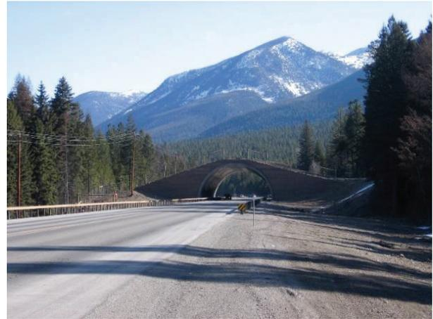
**FIGURE 24. US 93 WILDLIFE OVERPASS NEAR EVARO, MONTANA. PHOTO CREDIT: P. BASTING.**
