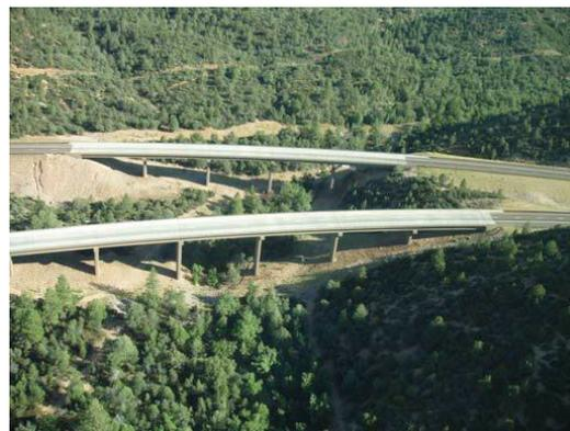
**FIGURE 53. TWO OF THE LARGE WILDLIFE CROSSING BRIDGES ON STATE ROAD 260, PAYSON, ARIZONA. PHOTO CREDIT: T. BRENNAN.**
