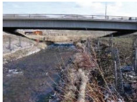
**FIGURE 31. THIS BRIDGE ON US 93 IN THE BITTERROOT VALLEY WAS LENGTHENED TO ACCOMMODATE WILDLIFE PASSAGE. PHOTO CREDITS: L. FRAZIER.**
