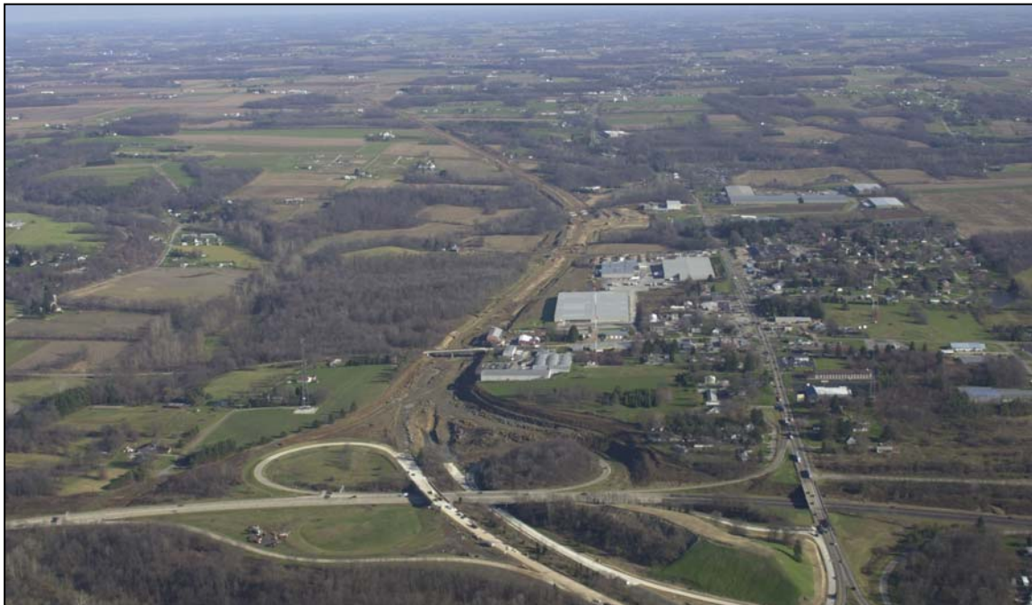
Figure 4. Aerial view of WAY30 test section location under construction.
