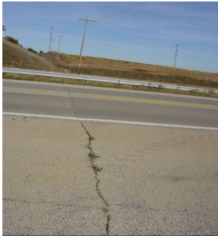
Figure E-1. Full-width thermal cracking
