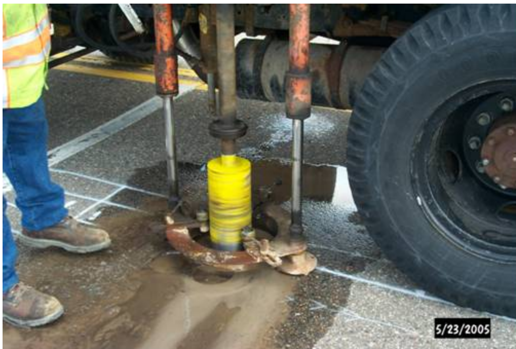
Figure C-2. Coring with core truck
