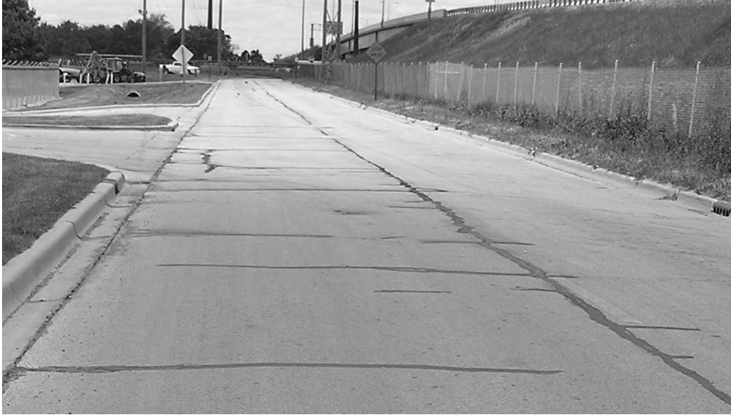
Figure 8.1. Observation of an asphalt overlay bonded to a base-layer with uniformly distributed cracks due to low temperature loading
