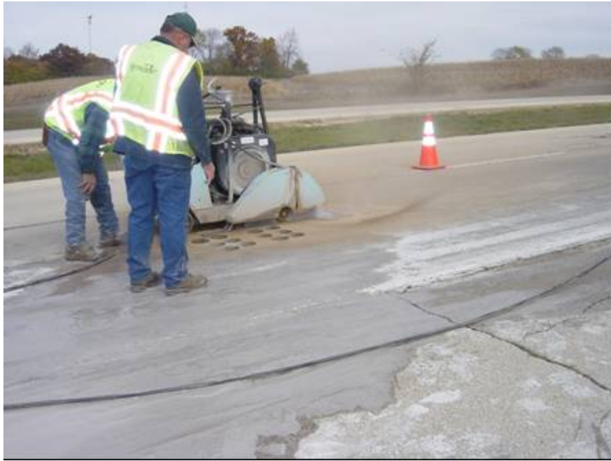
Figure D-4. Saw cutting
