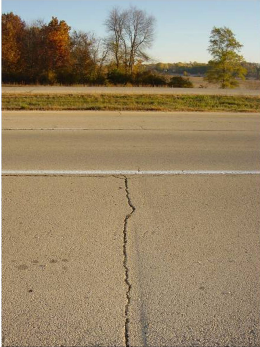
Figure E-2. Shoulder cracking
