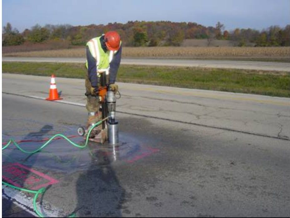
Figure D-2. Coring operation
