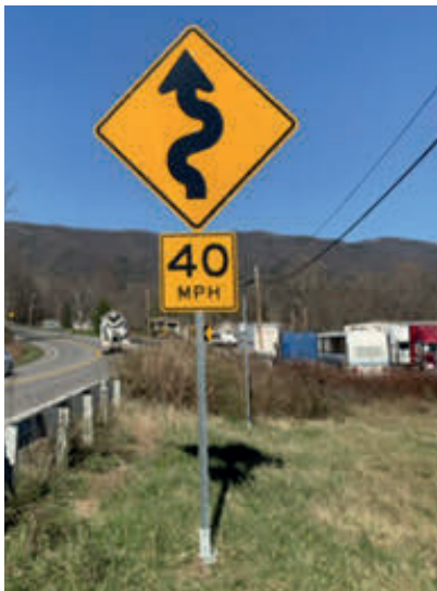
Figure 19. Photo. After treatment: oversized sign.
