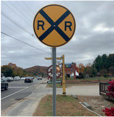
Figure 17. Photo. Before treatment: Railroad Crossing sign without retroreflective 2.5-inch yellow strip.
