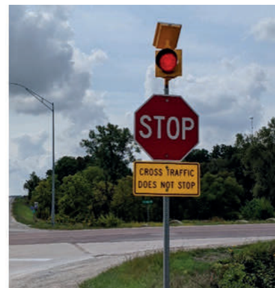
Figure 10. Photo. Treatment in Iowa: STOP-sign beacon.
