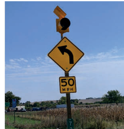
Figure 9. Photo. Treatment in Iowa: curve beacon.
