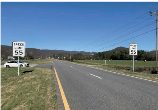
Figure 25. Photo. Conspicuity treatment: white retroreflective strip on signpost.
