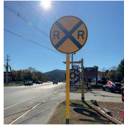
Figure 18. Photo. After treatment: Railroad Crossing sign with retroreflective 2.5-inch yellow strip.
