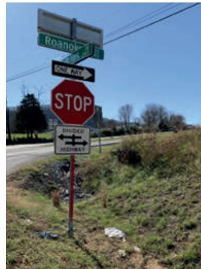
Figure 20. Photo. After treatment: red retroreflective strip.
