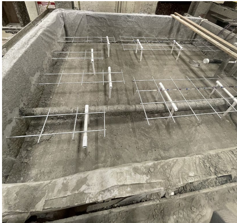
Figure 14. Photograph showing the welded-wire reinforcement layout for Test 7, with the left-hand side containing the reinforcements used for pull-out testing.
