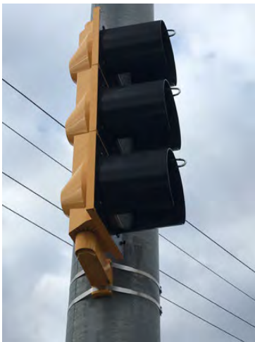
The installed new signals with a plastic weatherproof box for mounting the field monitoring system inside
