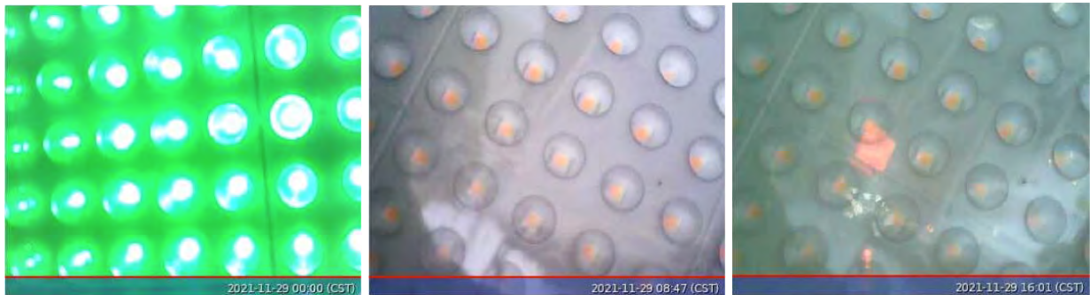
Figure 28: Wisconsin field test data collected in November 2021 after the field installation on November 3 rd , showing the normal performance of the red, yellow, and green signal lights under mild and cold weather conditions, especially for the green signal light which had the longest power-on time. Note that due to traffic control in the early morning before sunrise, the green signal light was remained always powered on at that intersection while red and yellow signals were rarely powered on, resulting in a large temperature gap between the green signal lens and the ambient air, with minimal heat buildup on the red and yellow signal lenses during the traffic control period (midnight - sunrise).
