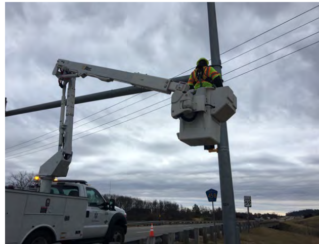
Remove the existing LED signals
