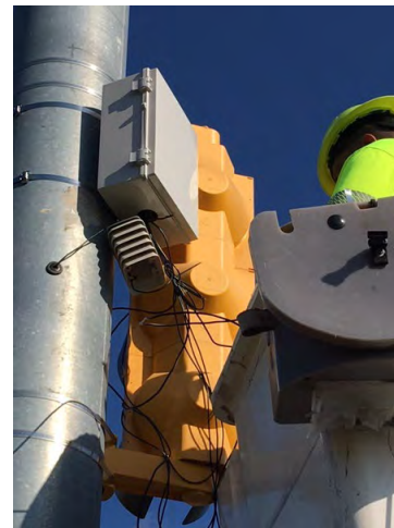
The installed new signals with a plastic weatherproof box for mounting the field monitoring system inside
