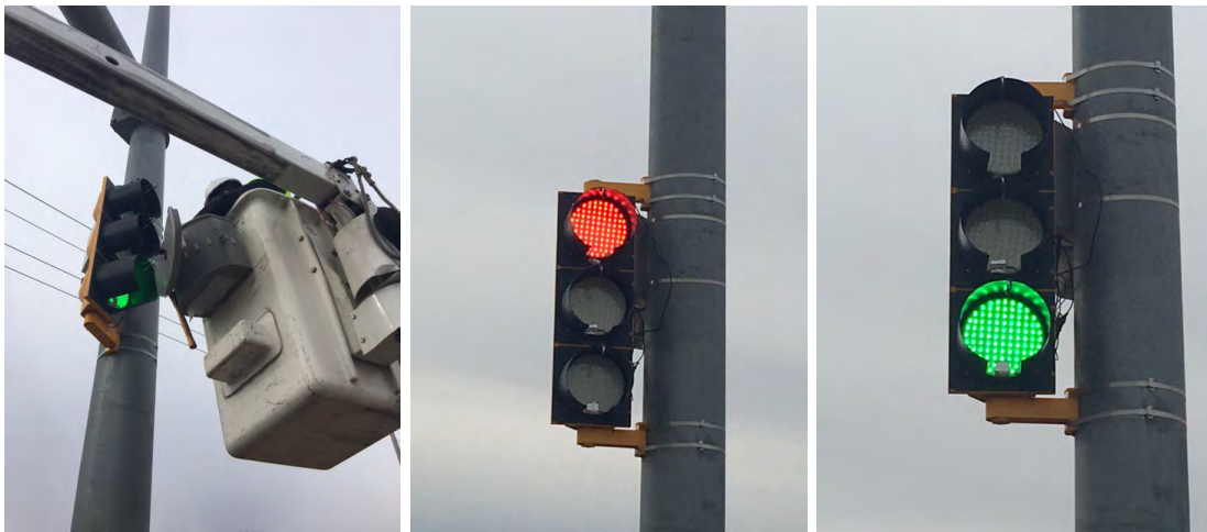
Figure 22: We stopped at the Lawrence field test site on Feb 25 th , 2021, with the Lawrence signal crew, to fix two problems related to the data collection and performance remote monitoring system (not part of the self-de-icing signal lights). We replaced the problematic cable cameras which failed after being exposed to the environment in the past two years, also fixed the loose mounting of the temperature sensors.
