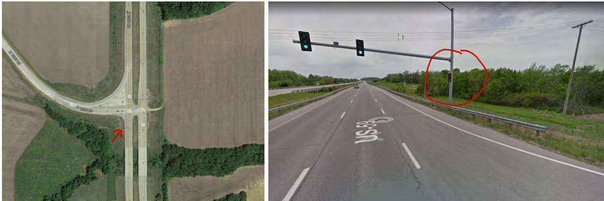
Figure 19: The first field test site in Kansas, at the intersection of County Rd 458 (or 1200 Rd) /US-59, where the selected signal head is on the right side of the road shoulder, facing north.
