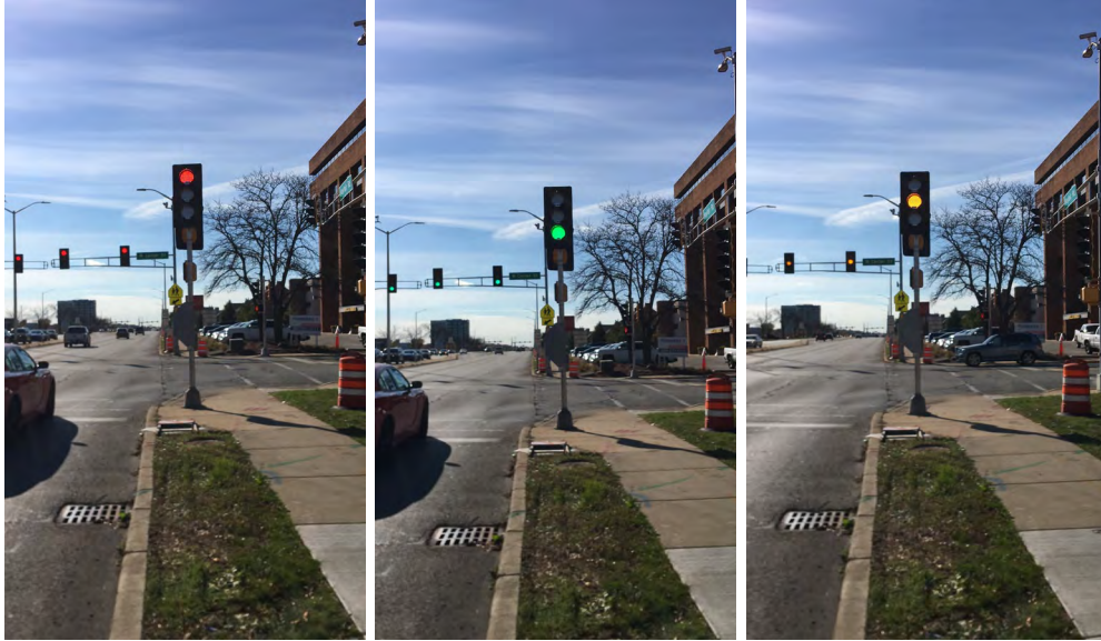
Figure 27: Field installation and setup of the onsite testing at the test site of Wisconsin, with the aid of the signal crew of Wisconsin DOT. A tunnel visor was installed with a hook for mounting the cable camera on each signal module. The signals are all facing north.
