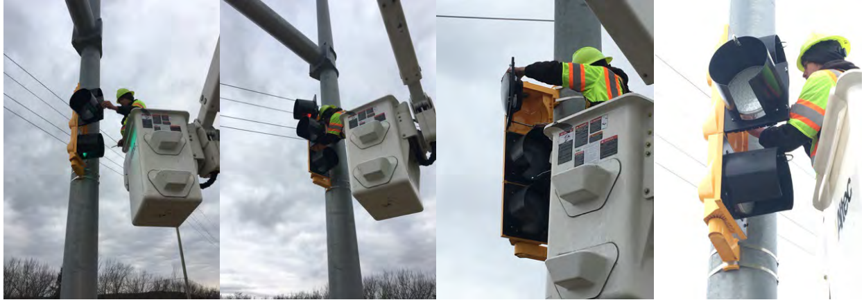
Replacing the old LED signals with the new self-de-icing signals
