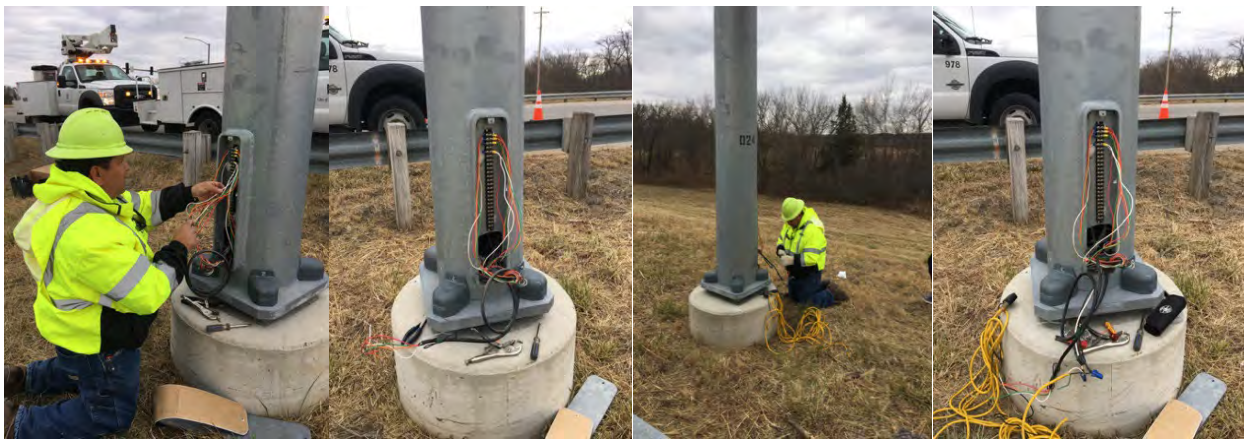
Wiring of the new signals
