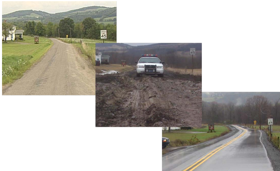
Figure 22. Roadway Impacts—Pavement to Mud and Then Restored.
