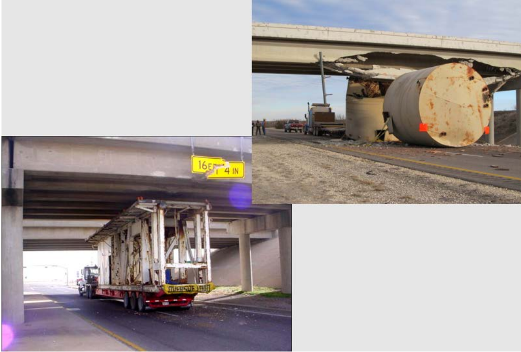
Figure 27. OS/OW Vehicles Hitting Bridges.
