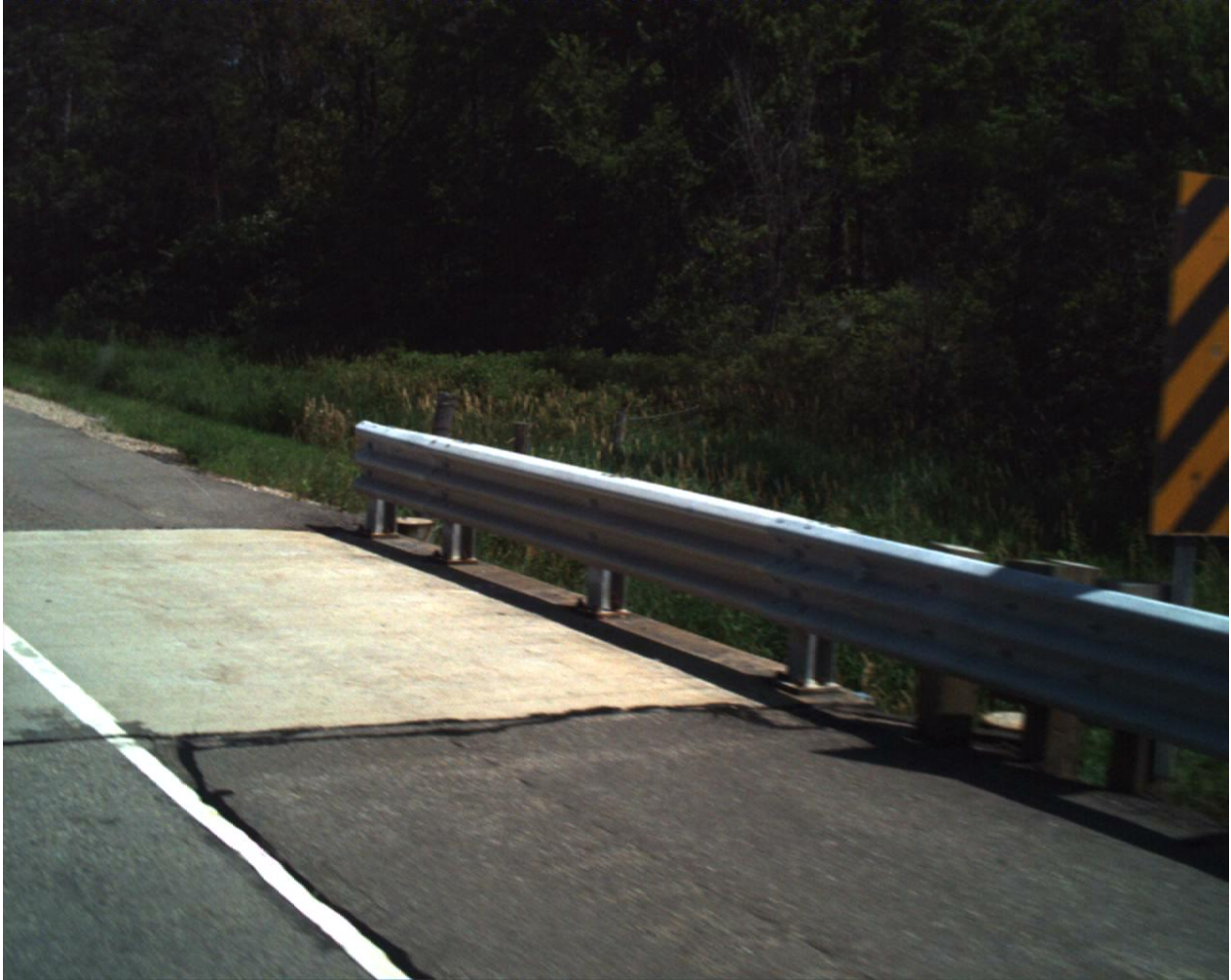
Figure 1. Thrie Beam Bridge Rail
