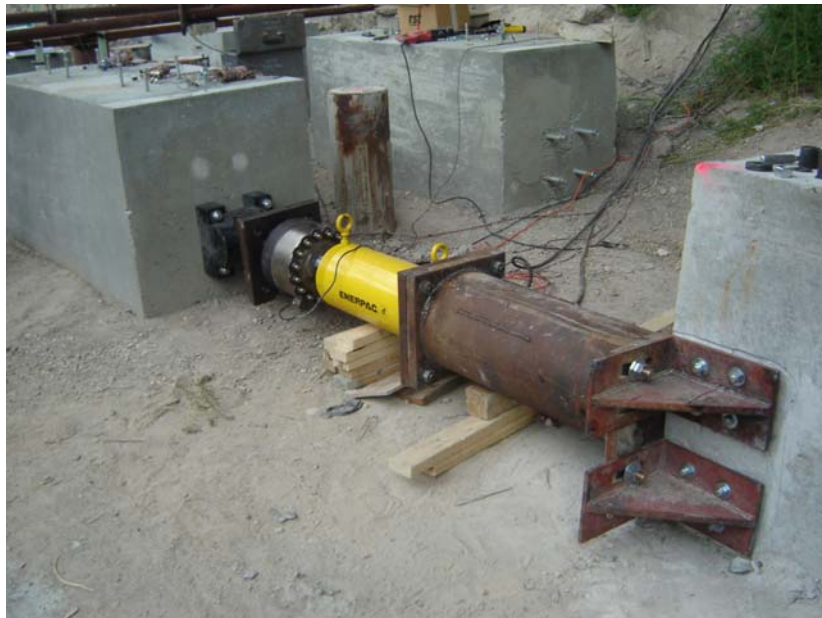
Figure 3 Pile cap test setup and with reaction provided by Geopier cap.
