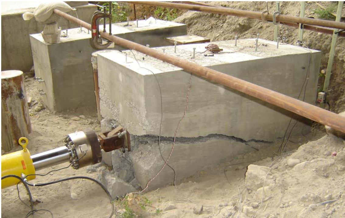
Figure 8 Failure of Test Cap 3.
