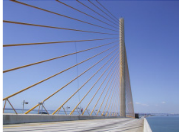
Figure 25: Stay and damper brace configuration.
