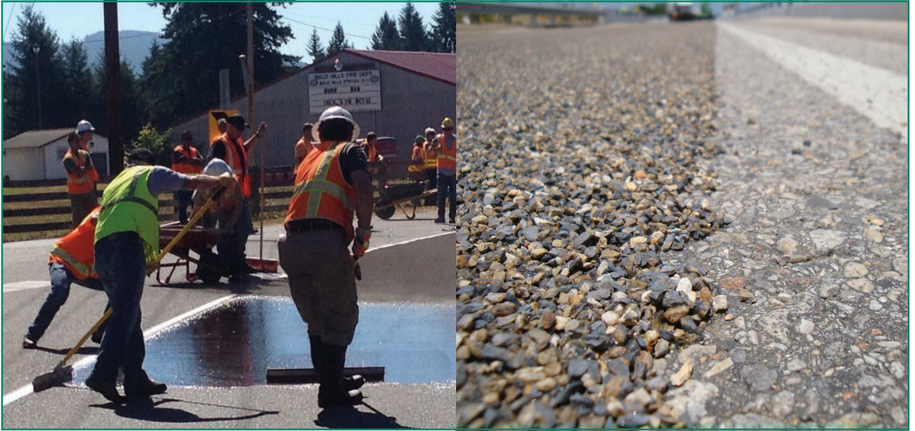
Source: FHWA. High-friction surface treatment has been shown to significantly reduce wet pavement crashes.
