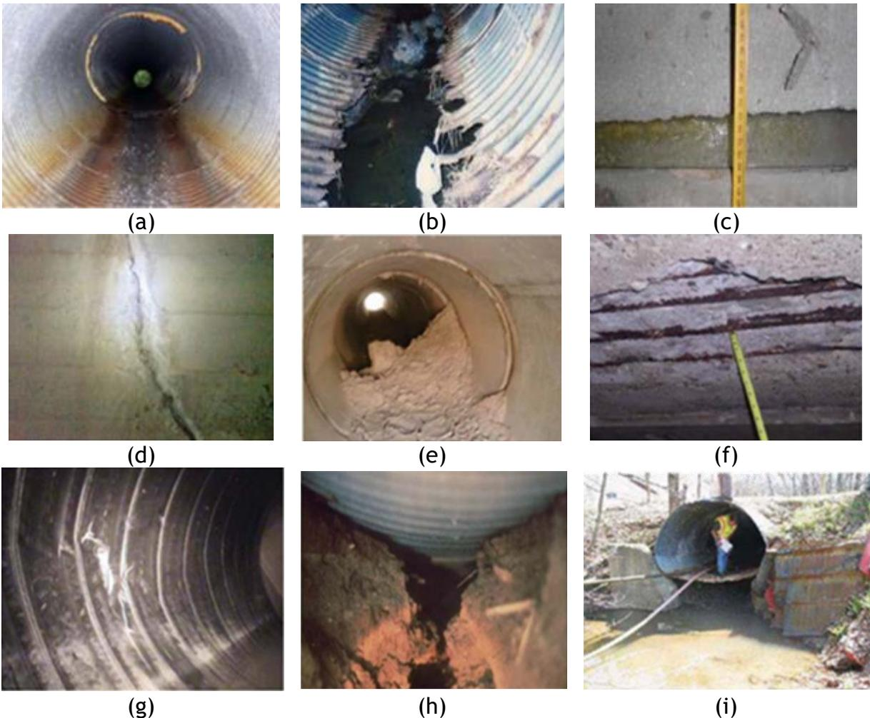
Figure 2-13. Common Defects of Culverts: (a) invert corrosion, (b) invert abrasion, (c) joint separation, (d) crack, (e) joint infiltration, (f) spalling in concrete culverts, (g) wall damages in plastic culverts, (h) piping beneath a culvert and (i) outlet scour (Piratla et al. 2017).
