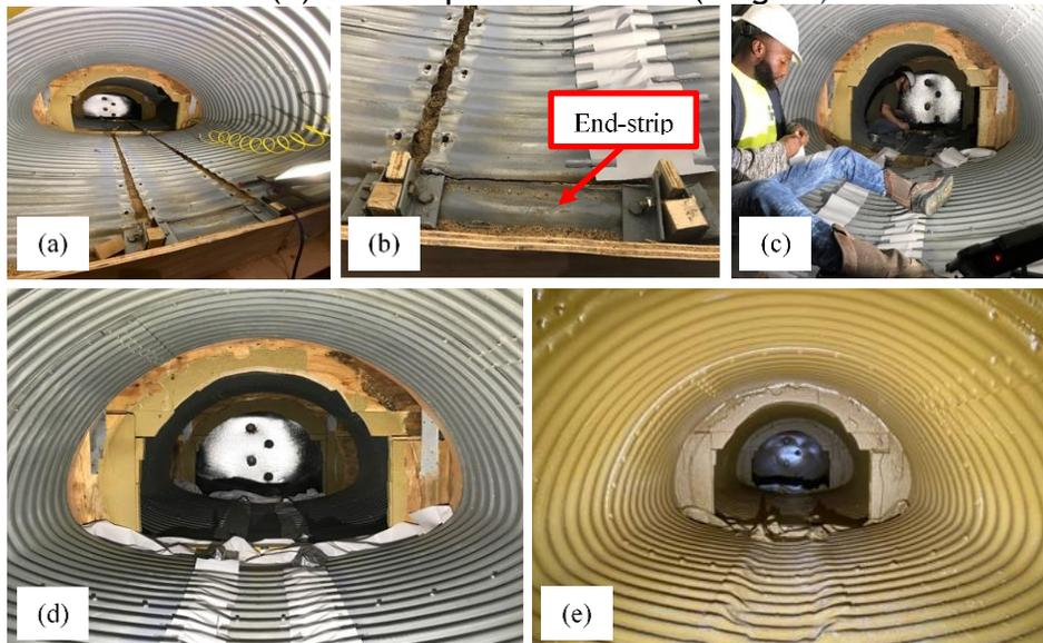
Figure 11-31. CMP arch preparation for SAPL installation: (a) CMP arch before gap sealing, (b) the invert-cut gap sealing with Styrofoam and plastic sheets, (c) Sprayroq's vendor working inside the CMP arch samples, (d) prepared pipe prior to the SAPL installation and (e) the SAPL renewed CMP arch samples.
