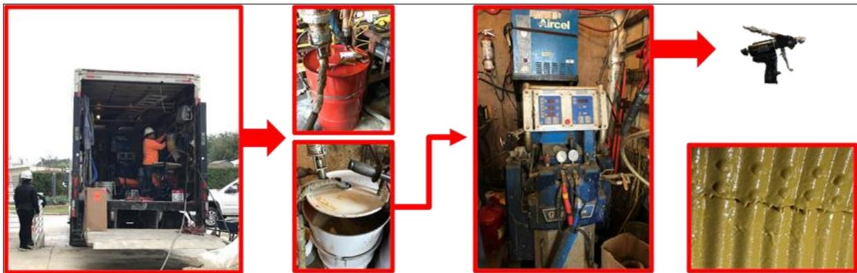
Figure 11-32. Hand spray SAPL installation.
