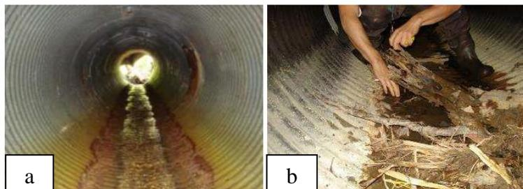
Figure 1. Structural condition of the culvert: (a) partially deteriorated and (b) fully deteriorated.
