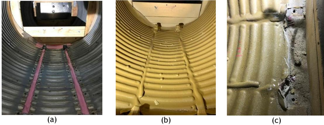
Figure 11-30. SAPL installation of invert-cut circular CMPs: (a) before SAPL installation (stage 1), (b) after SAPL installation (stage 2) and (c) end strips detachment (stage 3).
