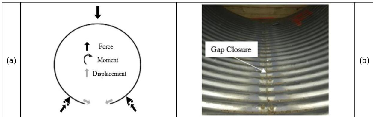
Figure 11-46. Circular CMP movement due to the invert detachment: (a) the movement mechanism, and (b) The gap closure at the cut location due to vertical loading.
