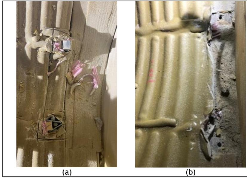
Figure 11-67. Invert-cut CMP arch end-strip detachment to remove the host pipe's ring stiffness: (a) over-sprayed SAPL and cutting process on the end-strip location, and (b) unbolted end-strip.
