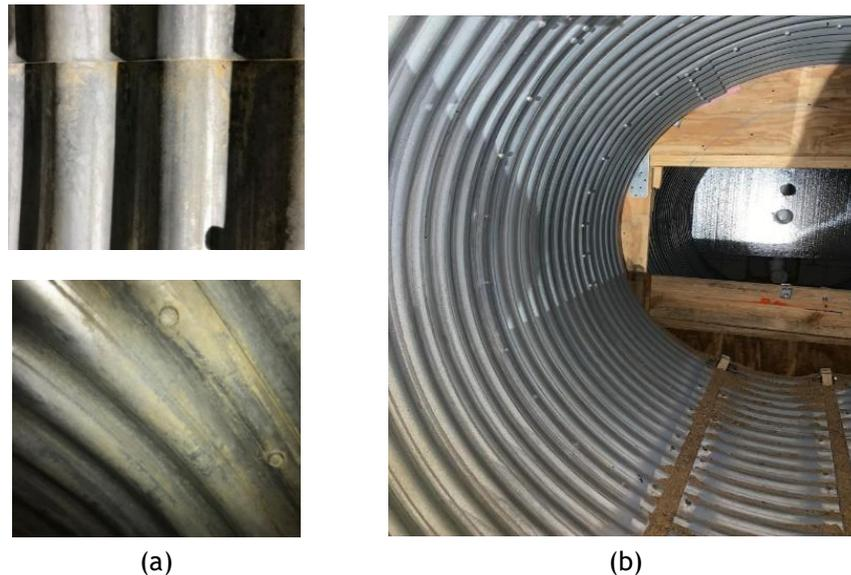
Figure 11-29. CMP surface preparation for SAPL installation: (a) dirt and dust on the CMP, and (b) CMP after power wash without any dirt and dust.
