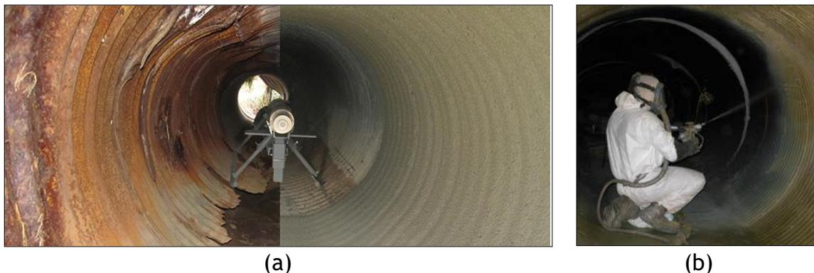
Figure 2-19. Corrugated metal pipe culverts (CMPs) before and after SAPL rehabilitation: (a) cementitious SAPL installation using spin casting machine (Source: CentriPipe) and (b) polymeric SAPL installation with hand spray (Source: Sprayroq).
