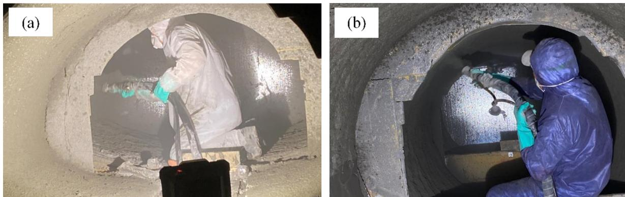
Figure 11-36. Cementitious SAPL installation on: (a) CMP arch and (b) circular CMPs.
