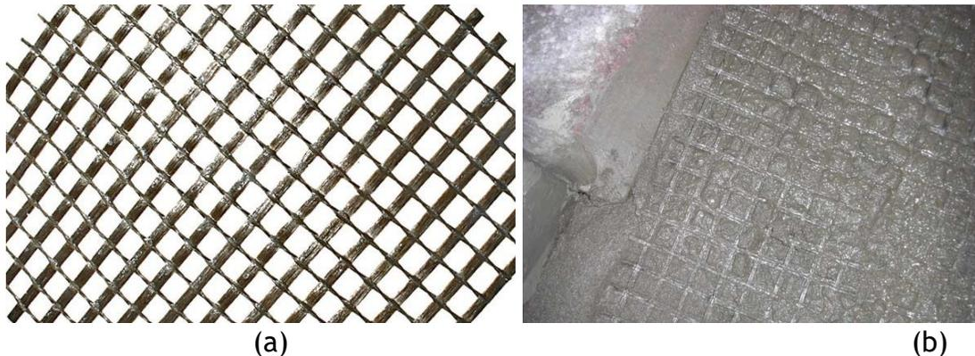
Figure 3-6. (a) Basalt Mesh Grid with 10 mm by 10 mm Opening, (b) Basalt Mesh Placed into Wet Concrete Prior to Final Layer's Placement.
