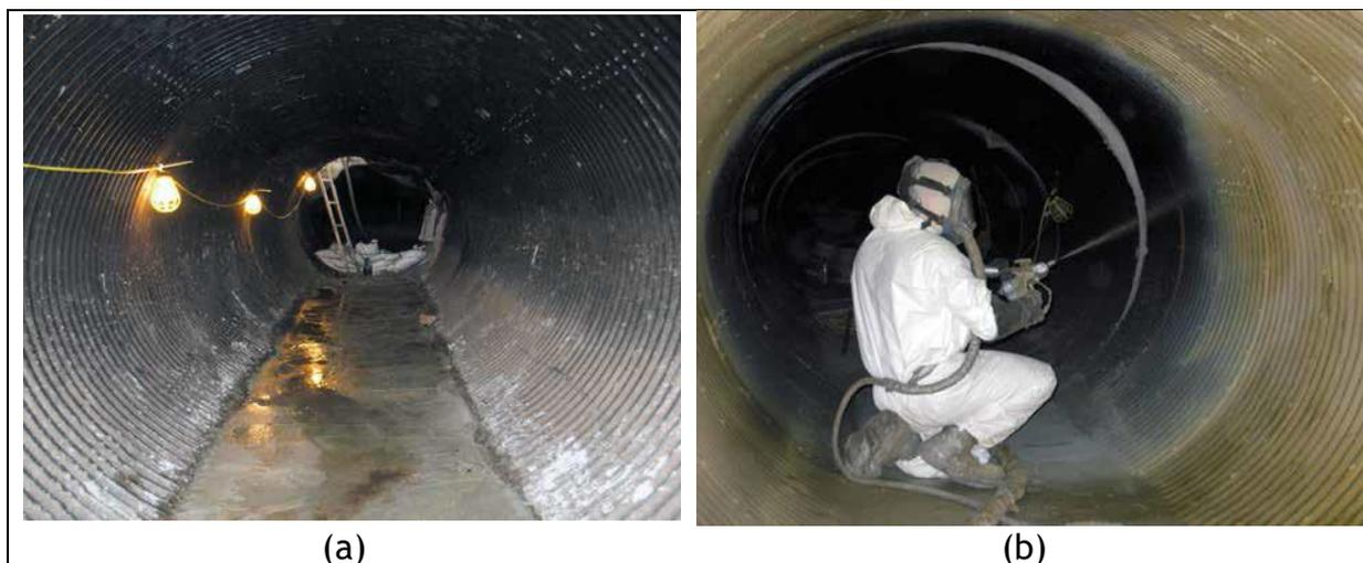
Figure 2-23. CMP renewal using SprayWall® polyurethane SAPL, Norristown, PA:
