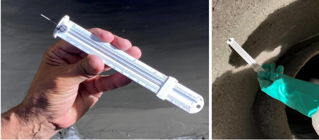
Figure 11-37. Thickness measurement using a depth gauge at the time of SAPL installation.
