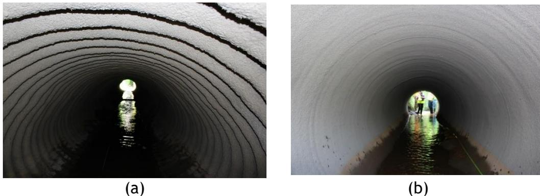
Figure 5. Two common SAPL installation methods: (a) following and (b) filling the corrugation pattern.
