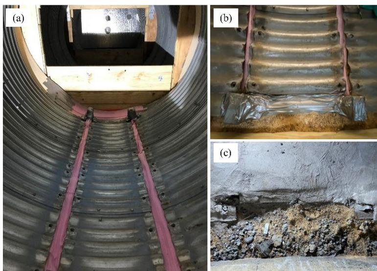
Figure 11-35. End-strip detachment: (a) end-strip preparation, (b) end-strip before SAPL installation and (c) end-strip detachment after SAPL installation.
