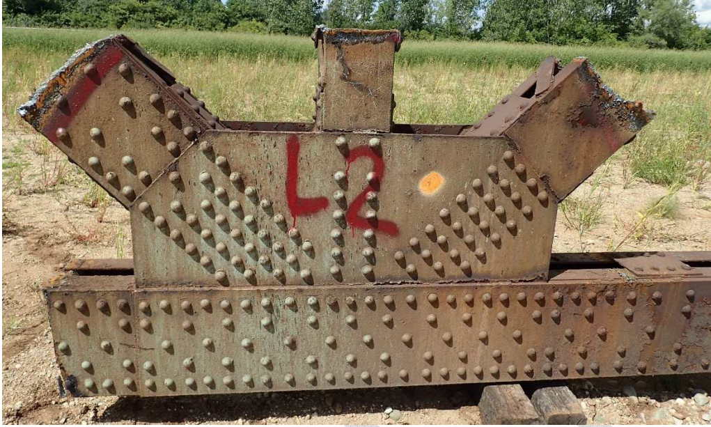
Figure 4.46 Example of deeply set two-channel diagonal members connected into a gusset plate
