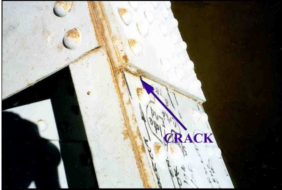
Figure 2.2 Fractured tie girder plate, Hastings Bridge (Niemann, 1999)
