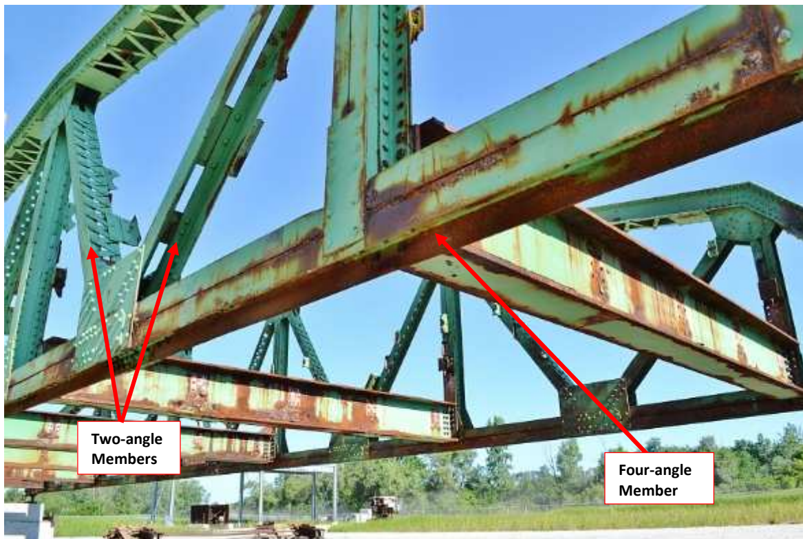
Figure 4.20 Simple-span pony truss showcasing several angle-only member types
