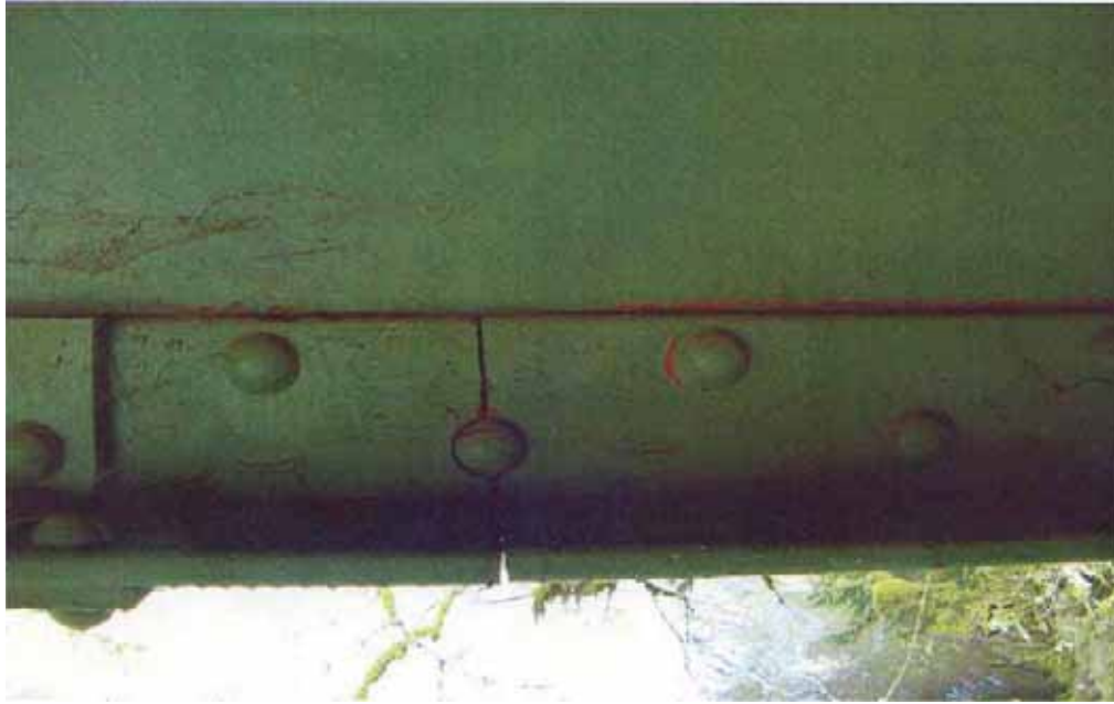
Figure 2-2 Interior view of fractured flange angle (Lovejoy, 2001)
