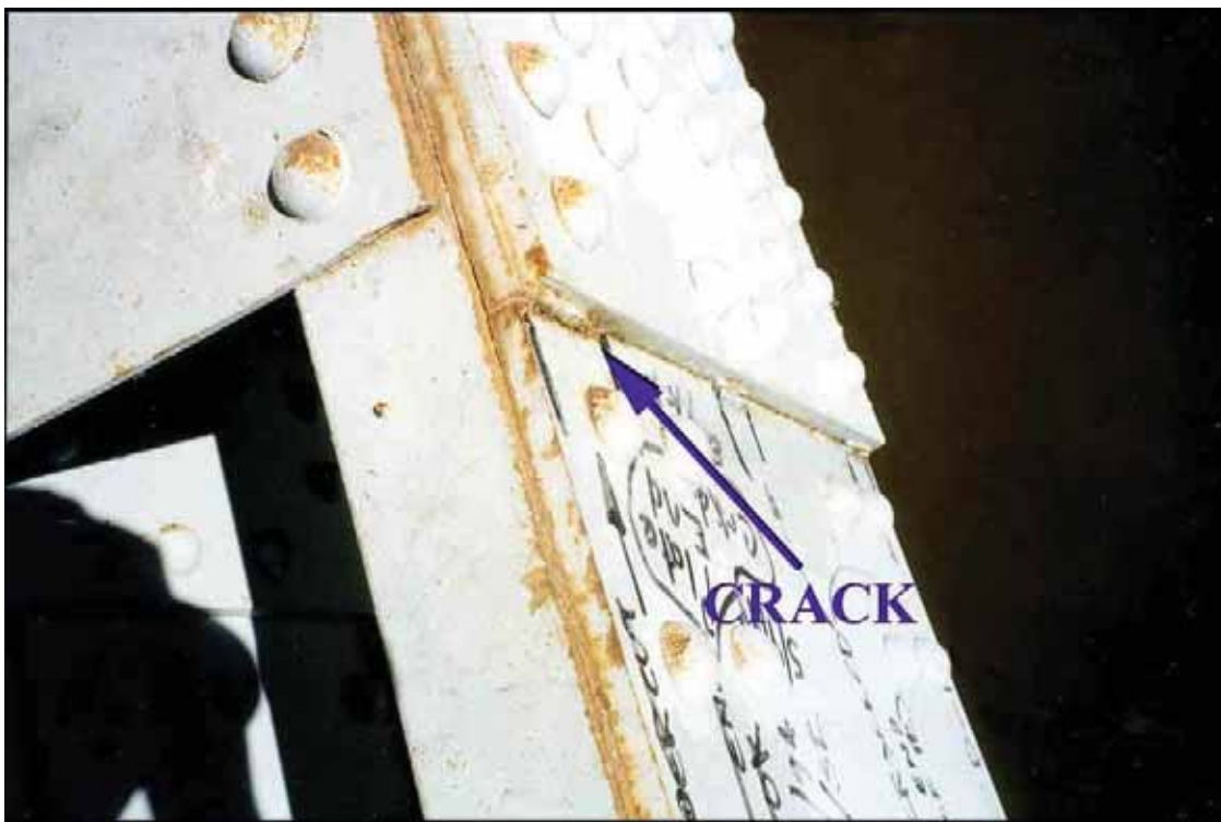
Figure 2-6 Fractured tie girder plate, Hastings Bridge (Niemann, 1999)
