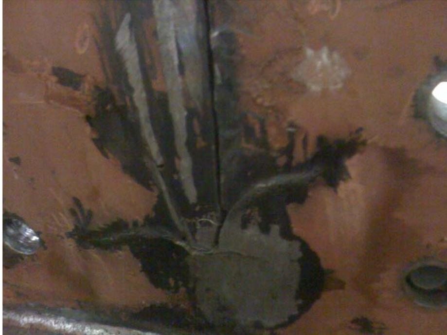
**Figure B.66: Existing cracks on exterior face of the girder's web**
