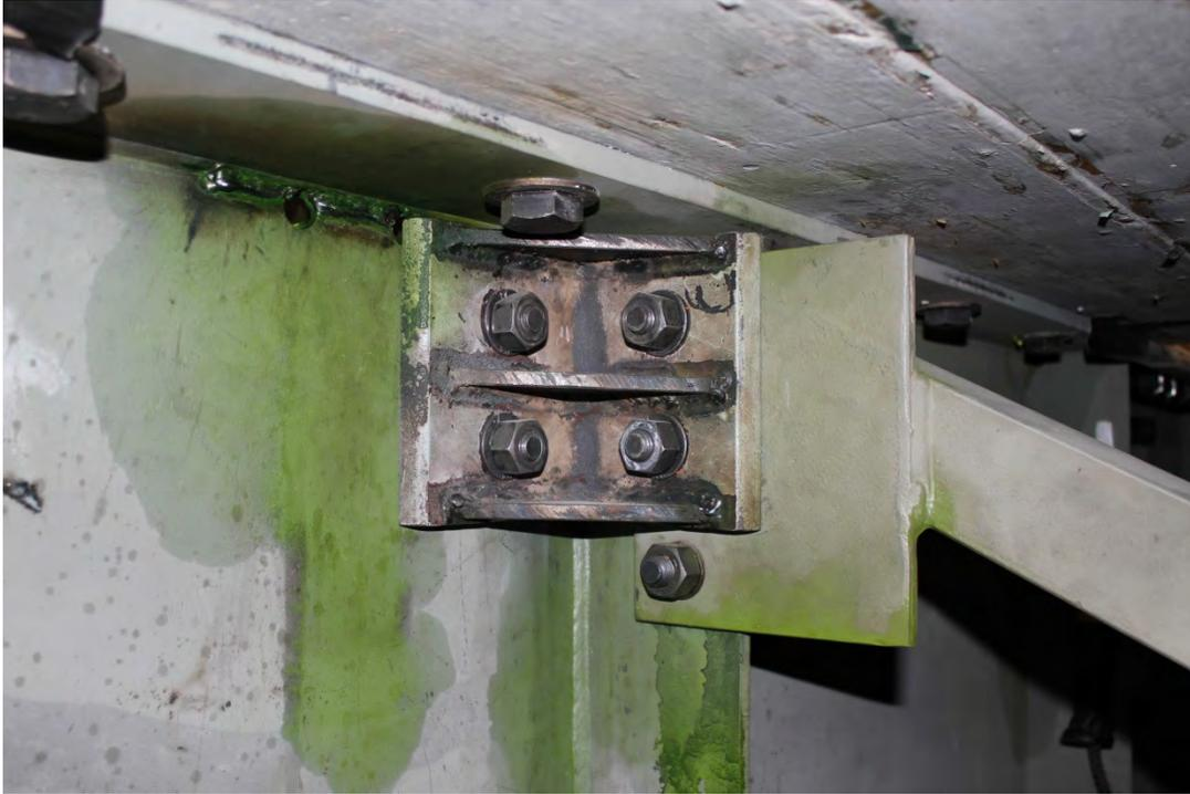
**Figure A.26: Stiffened angles-with-plate retrofit applied to exterior girders in Trial 7**
