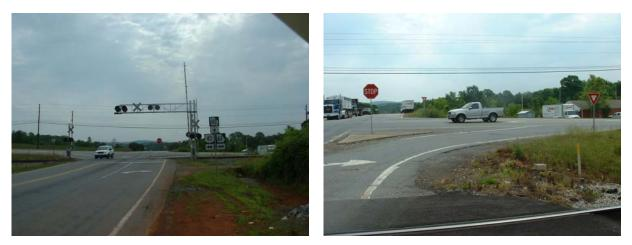
**FIGURE 4-8** GA 140 Eastbound Approach (left photo) and Channelized Right Turn Lane (right photo)
