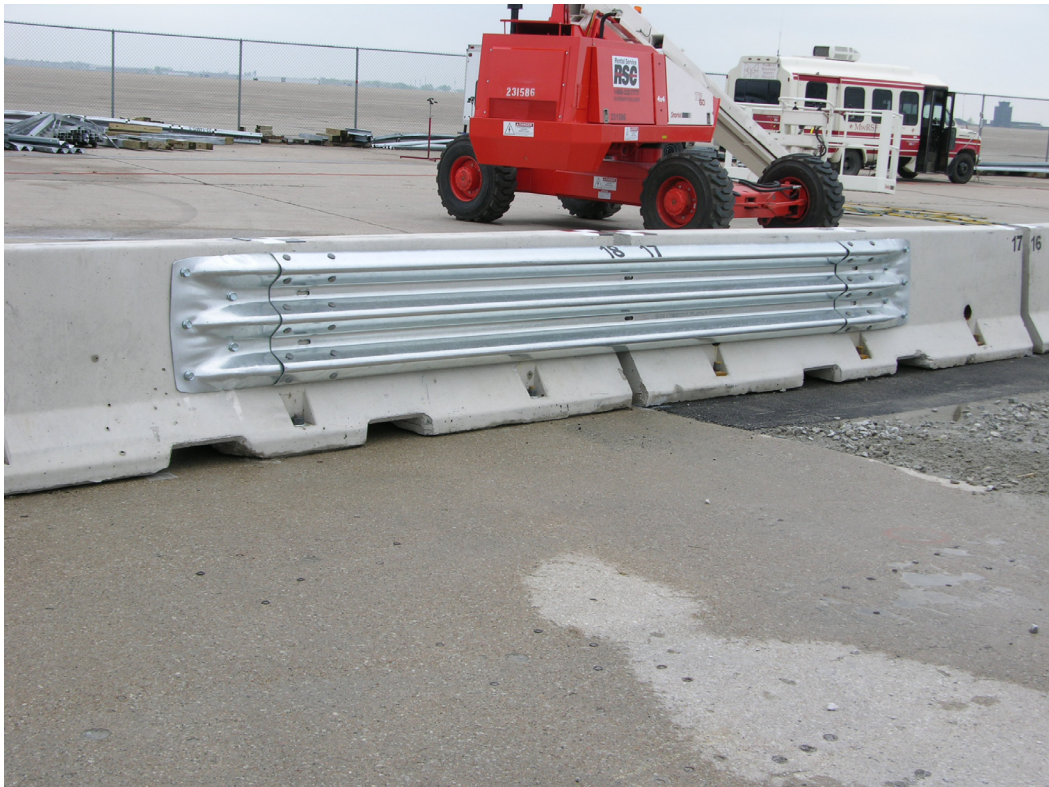
Figure 46. Free-Standing to Rigid Concrete Barrier Transition Photographs
