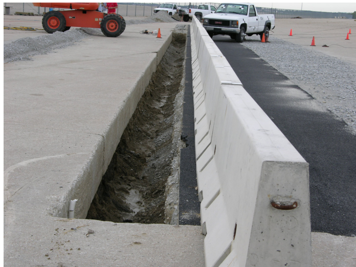
Figure 12. Asphalt Pin Tie-Down Design Photographs
