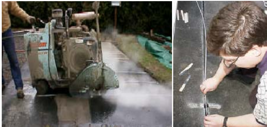
Figure 5.14. Installation of the Long Gage FBG Sensors.
